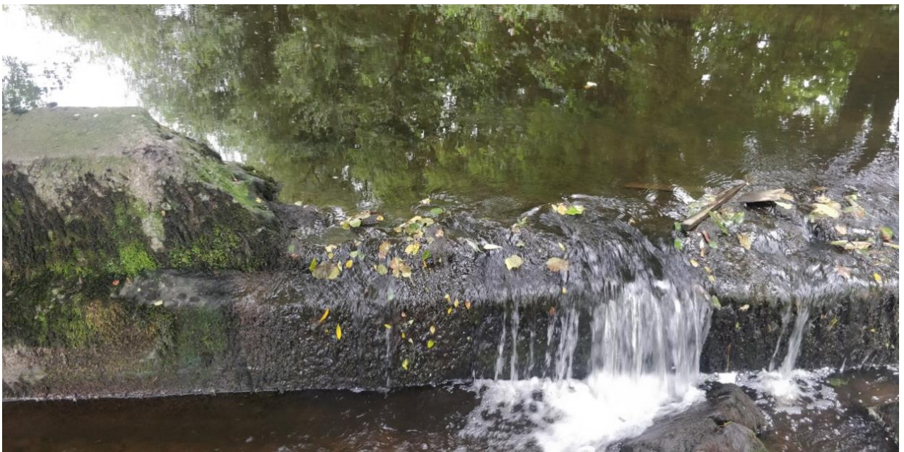
Figure 3. The weir is constructed from concrete.
