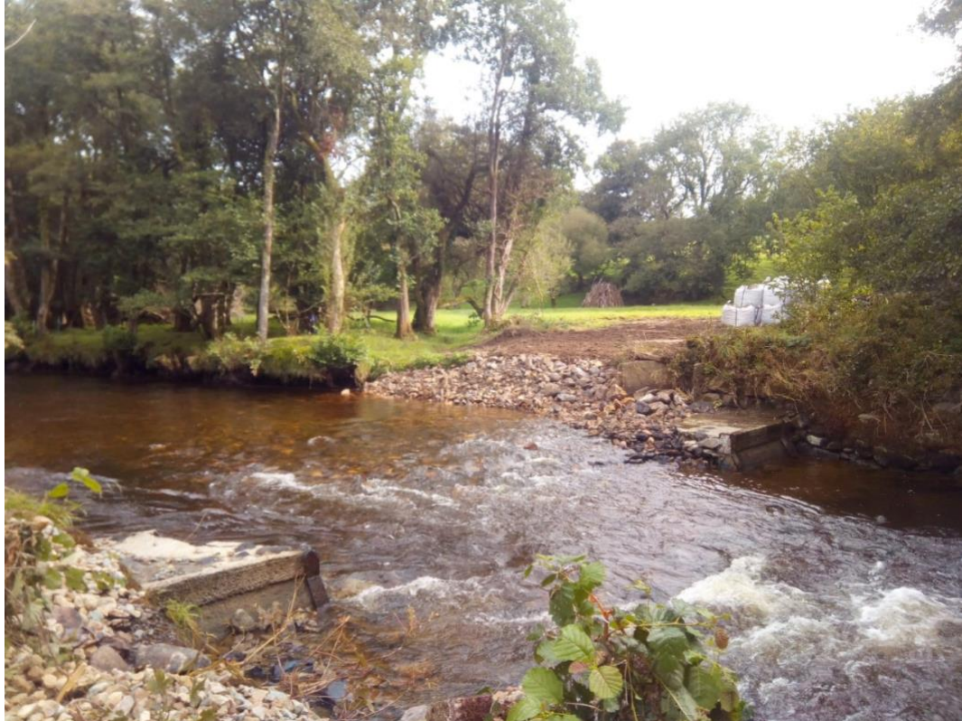
Figure 10. Example of riprap used to protect bankside and gain working entry to the river.
