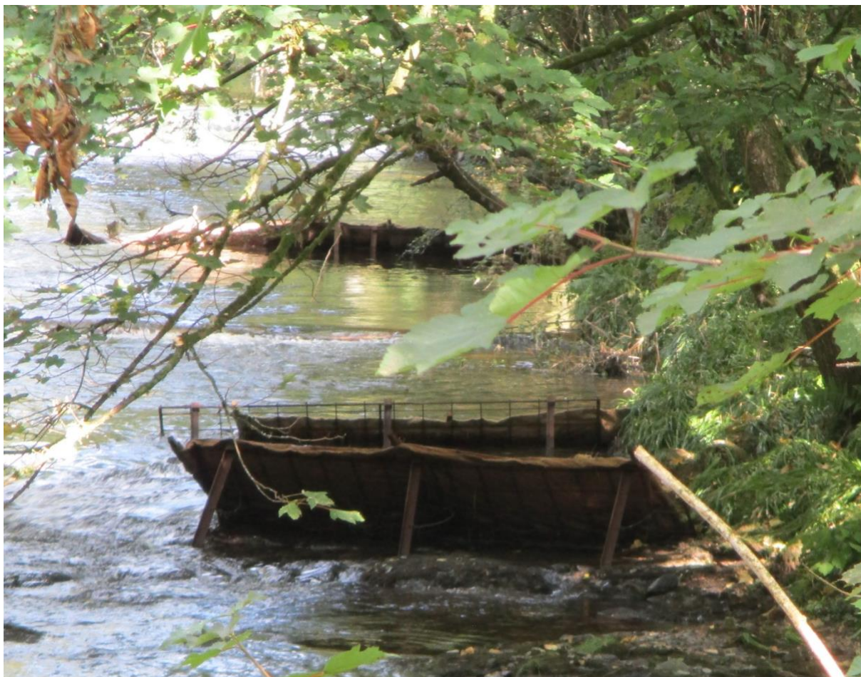
Figure 8. Sedimats installed within the river.
