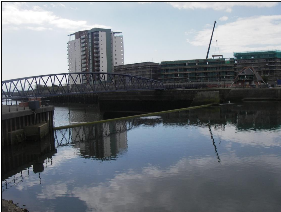
Figure 1.1 – The Tawe Barrage with the inlet to the hydrogenerator shaft in the foreground
