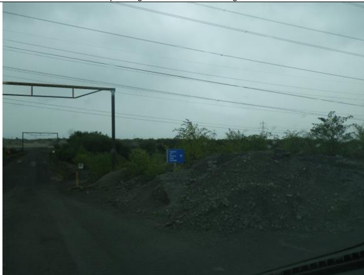
Photo 128 – Power lane valley looking towards BFS East and Lagoon 25
