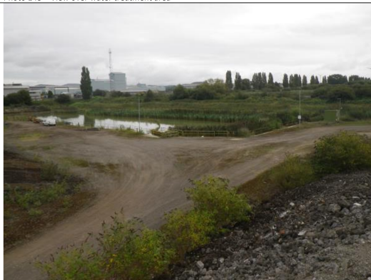
Photo 143 – View over water treatment area
