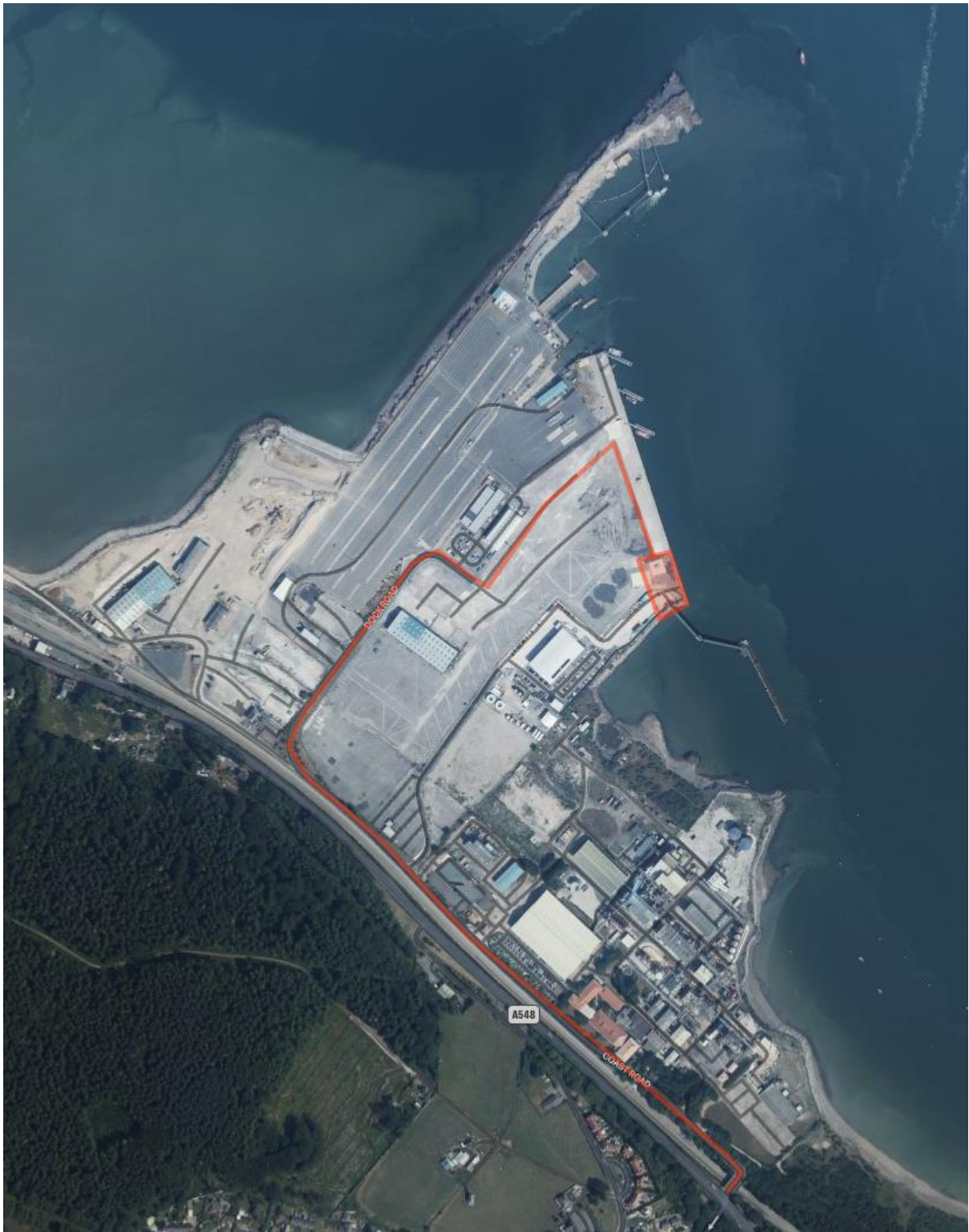
Port of Mostyn site access/egress and working area.
