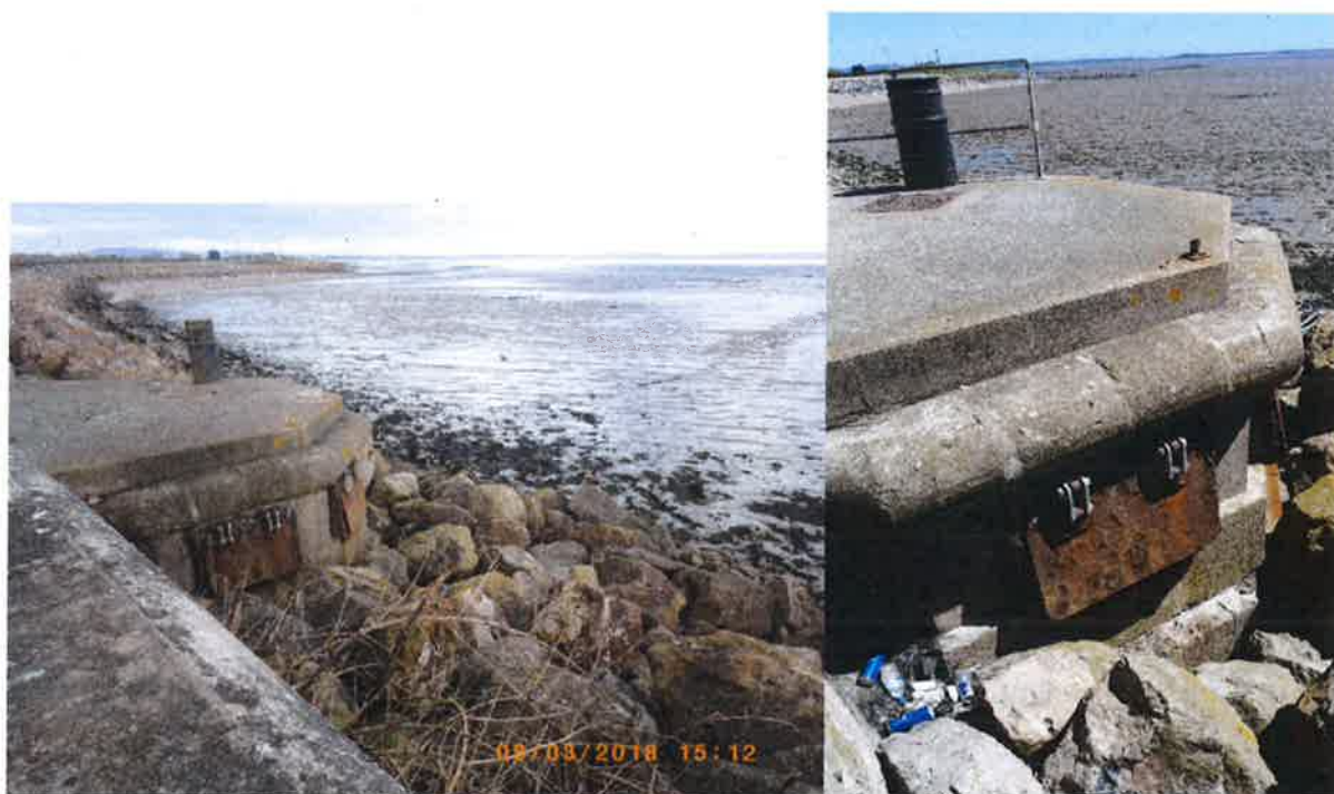
Figure2- Image of sea bound outfall structure and external flap valve arrangement
