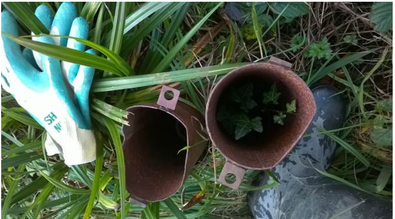
Photo 2 showing an open gas monitoring point with ivy inside security cover
