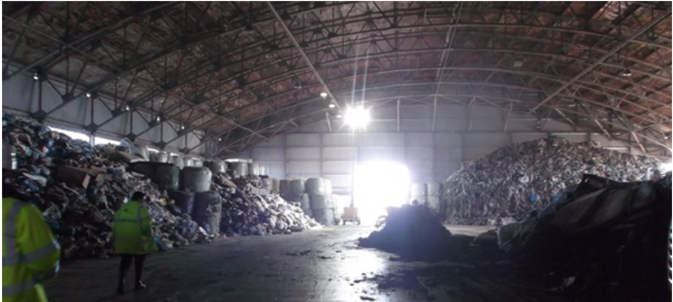
Waste stockpiles within Hangar B
