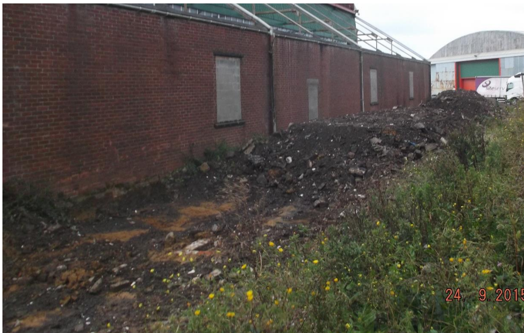
Picture of the soils contaminated with mixed waste from the old MRF excavated and pulled back
