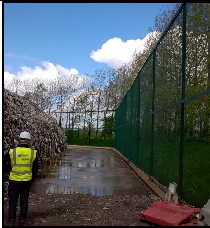
Picture 3 – taken on 02/05/18, showing five metre mesh fencing installed around the loose shredded material stored on impermeable surface near the transfer station
