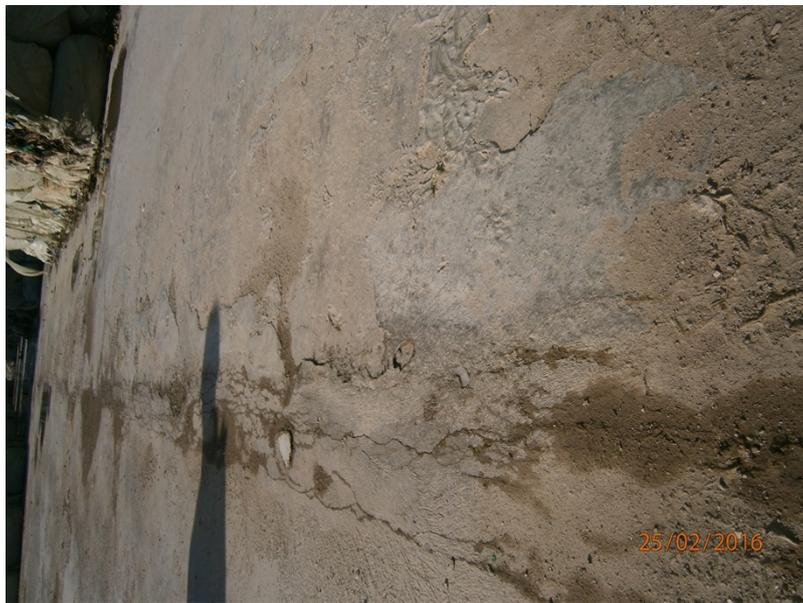
The images above are examples of the surface being not fit for purpose and therefore not compliant with the permit conditions. There has even been cracking taking place post repair work as can be seen clearly.
