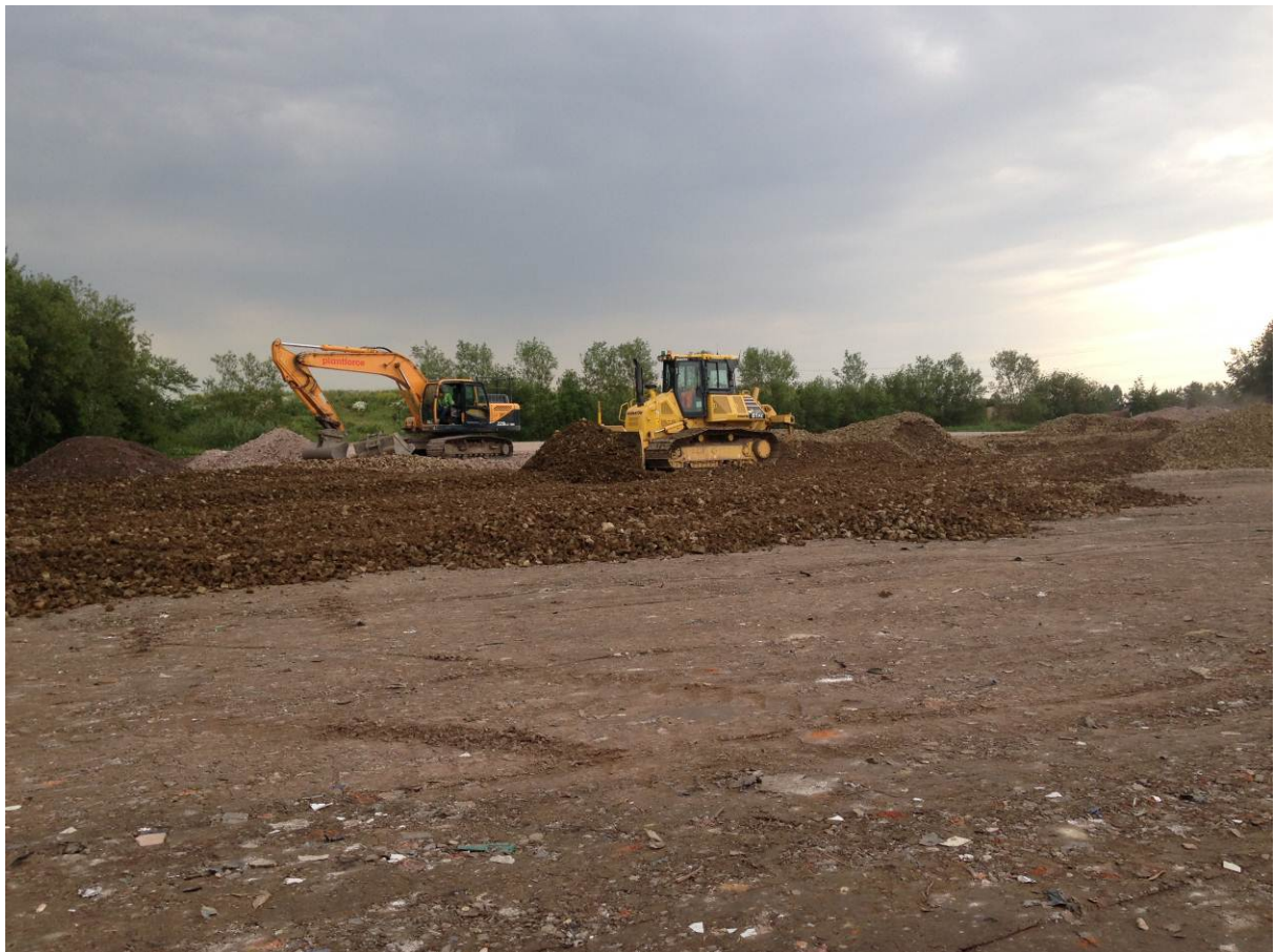
Placement of 200mm thick layer
