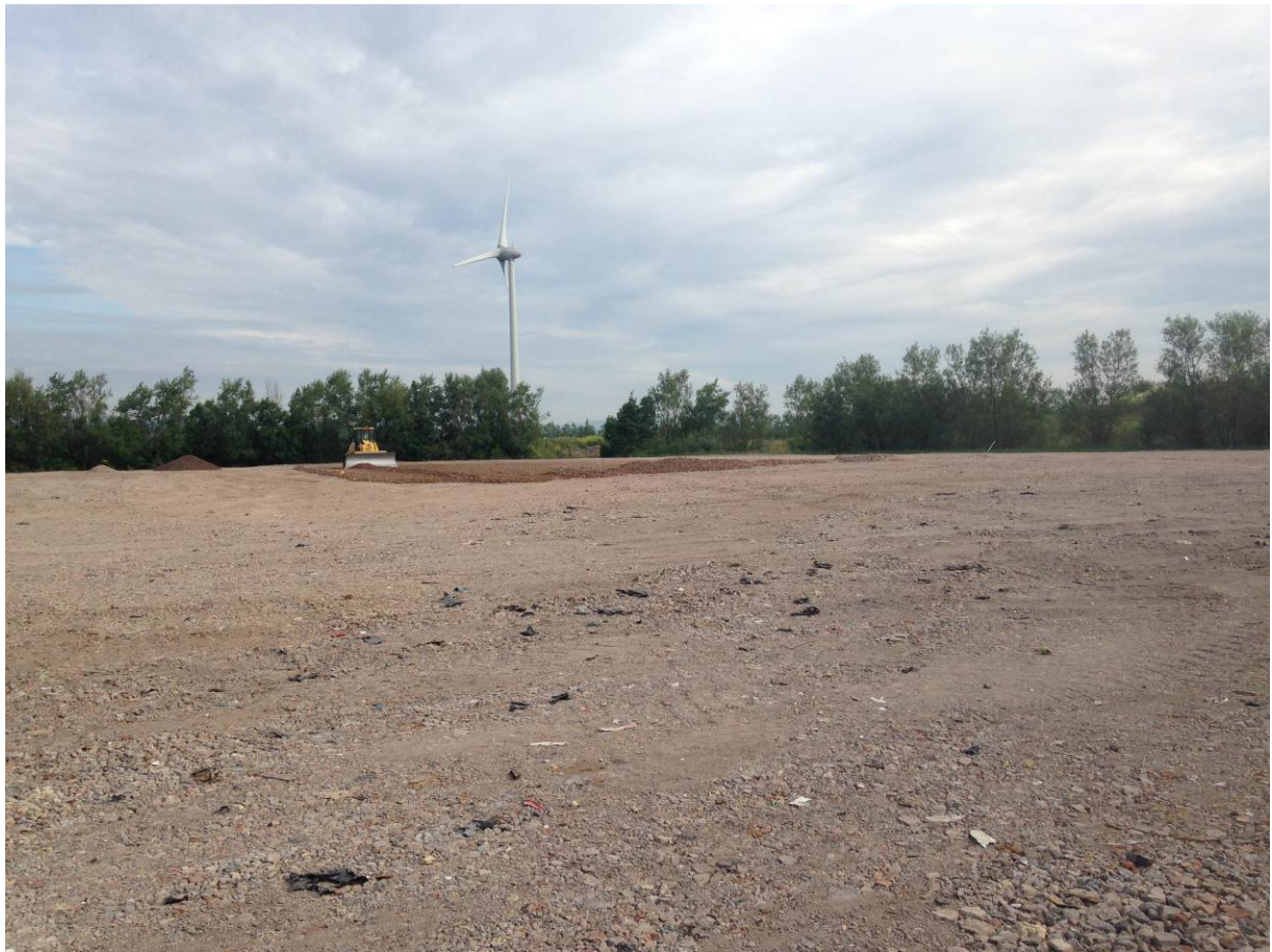
Final grading of surface with fine aggregate
