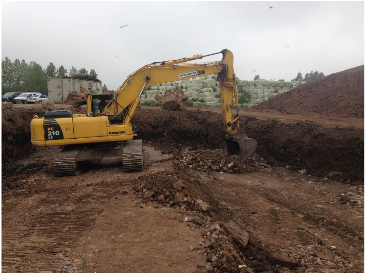
Removal of soft natural ground
