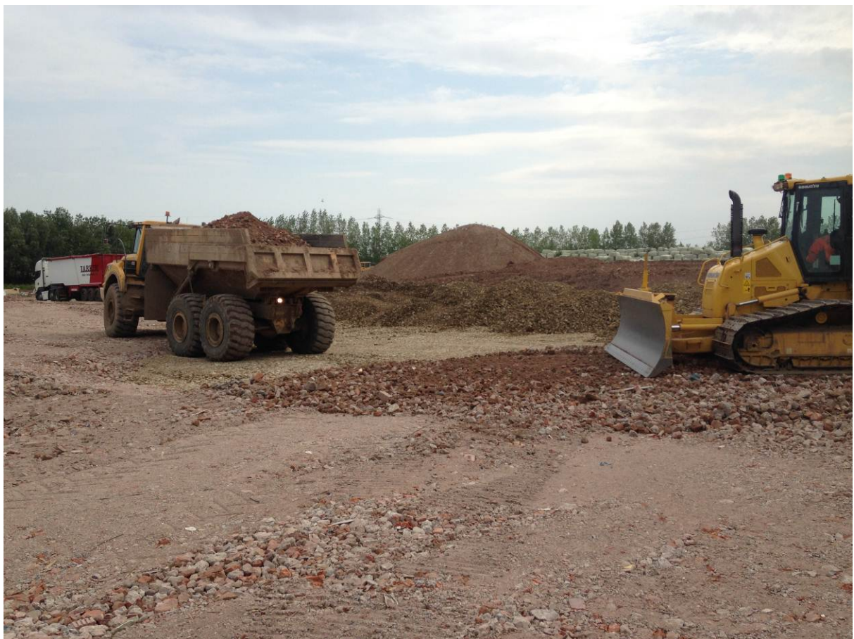
Delivery and spreading of aggregate
