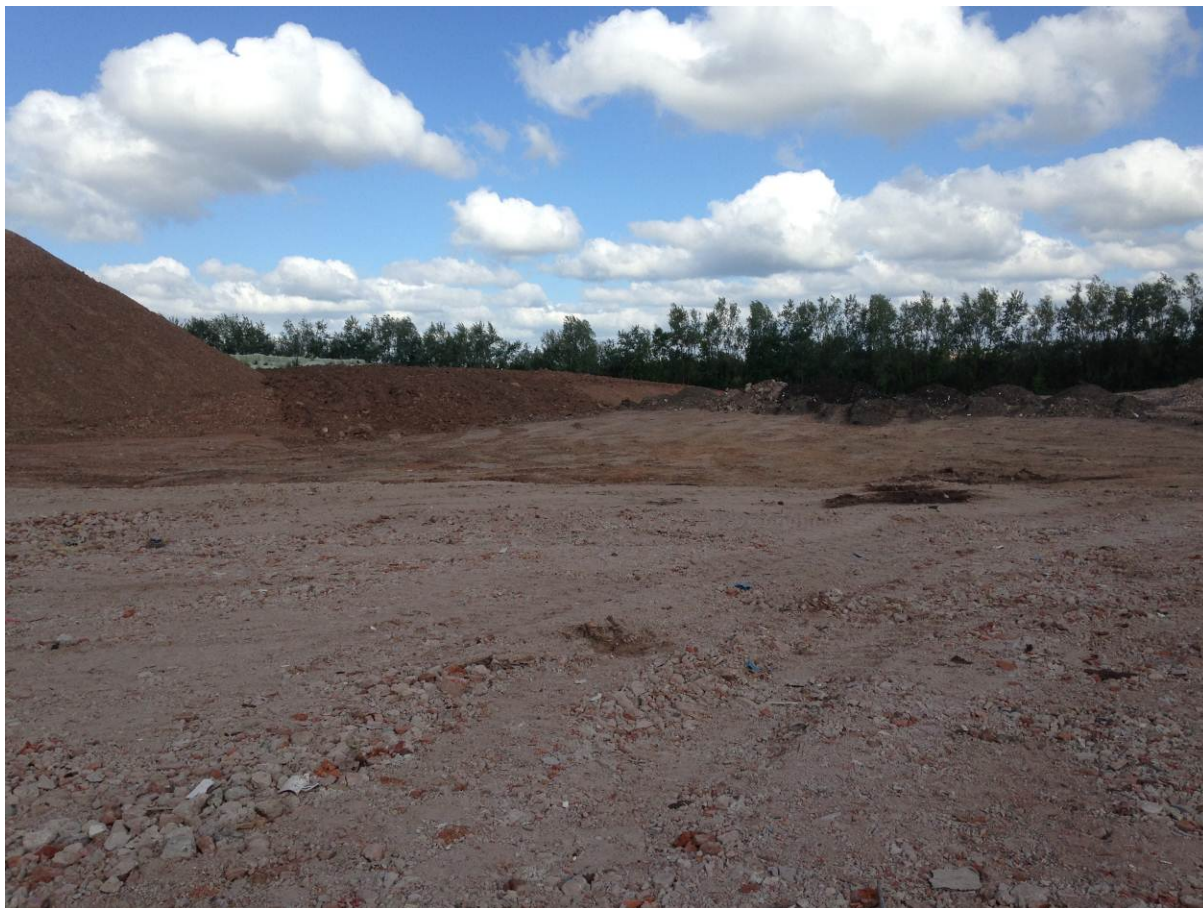
Ground condition prior to works
