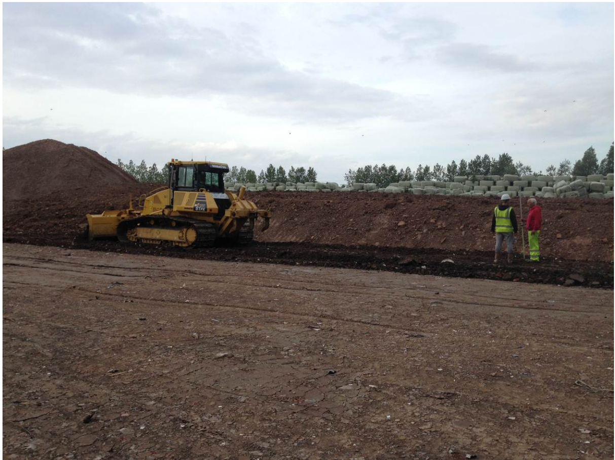
Level checks with grading laser
