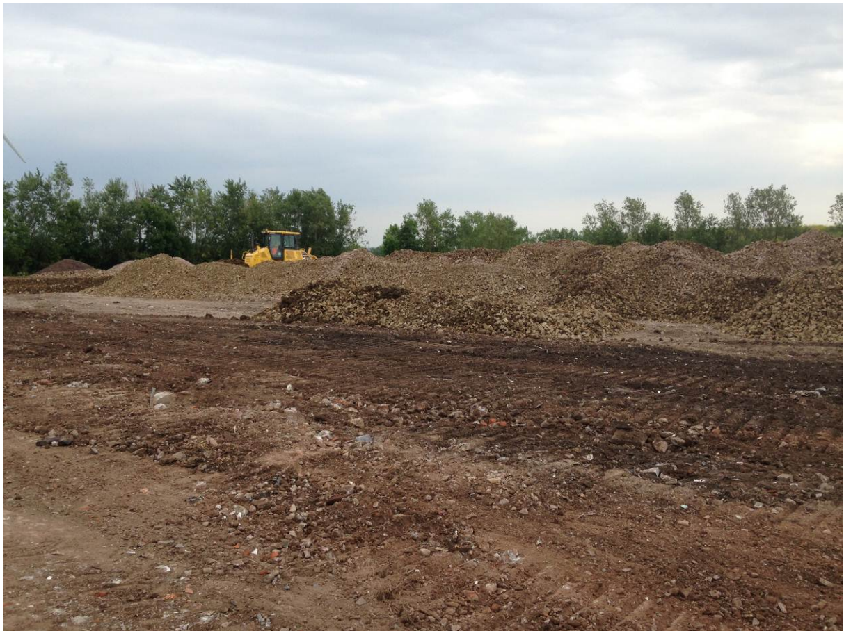
Formation and spreading of 200mm thick aggregate layer
