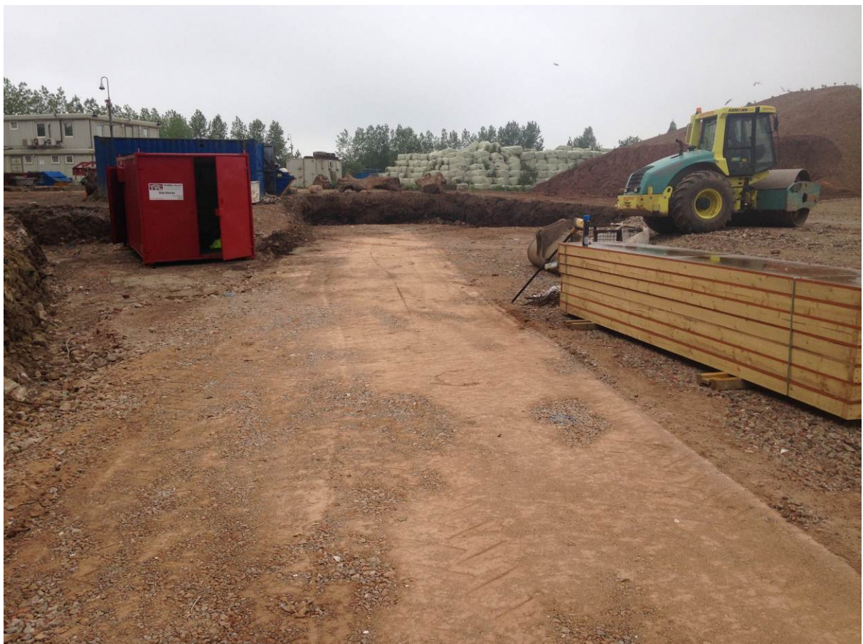
Reinstated area with dust finish for concrete
