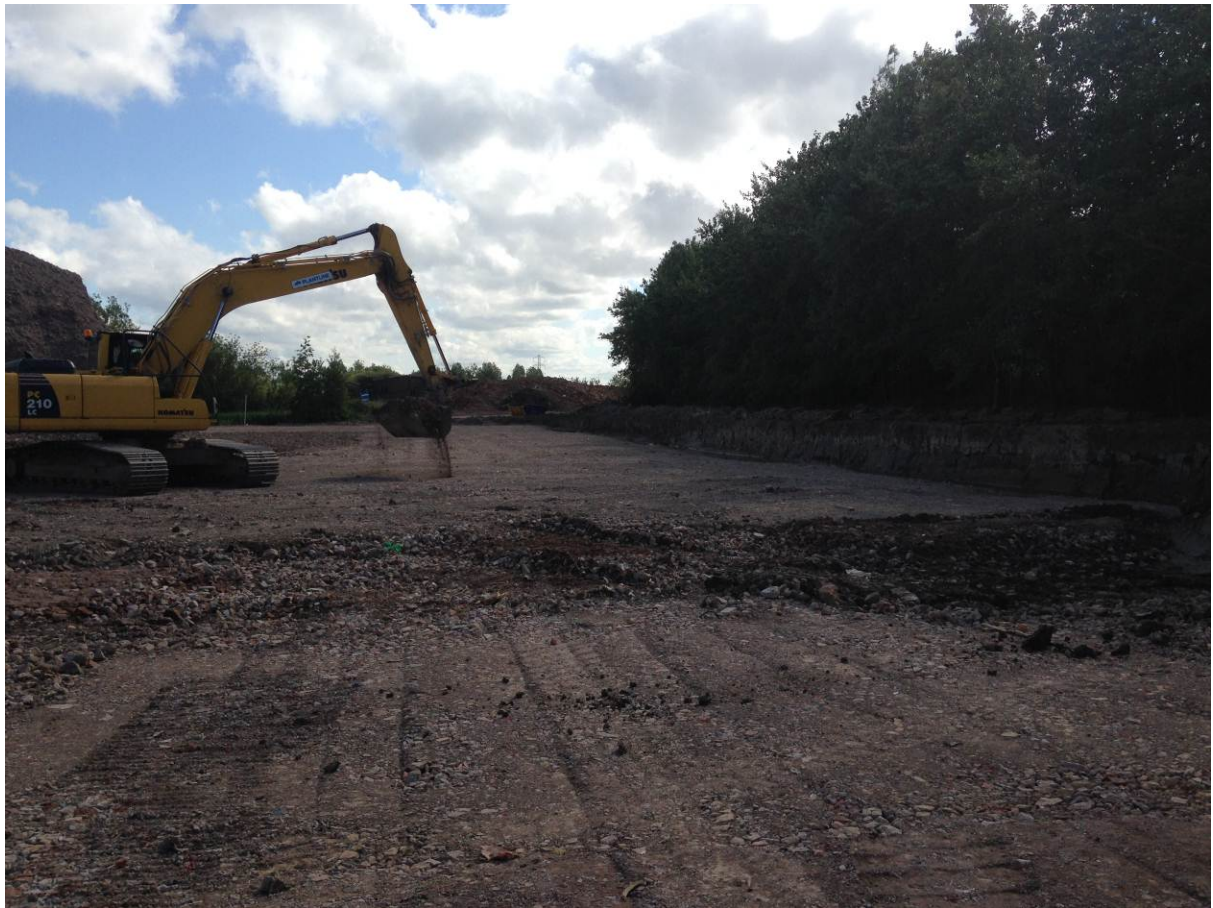
Placement of 200mm thick aggregate layer
