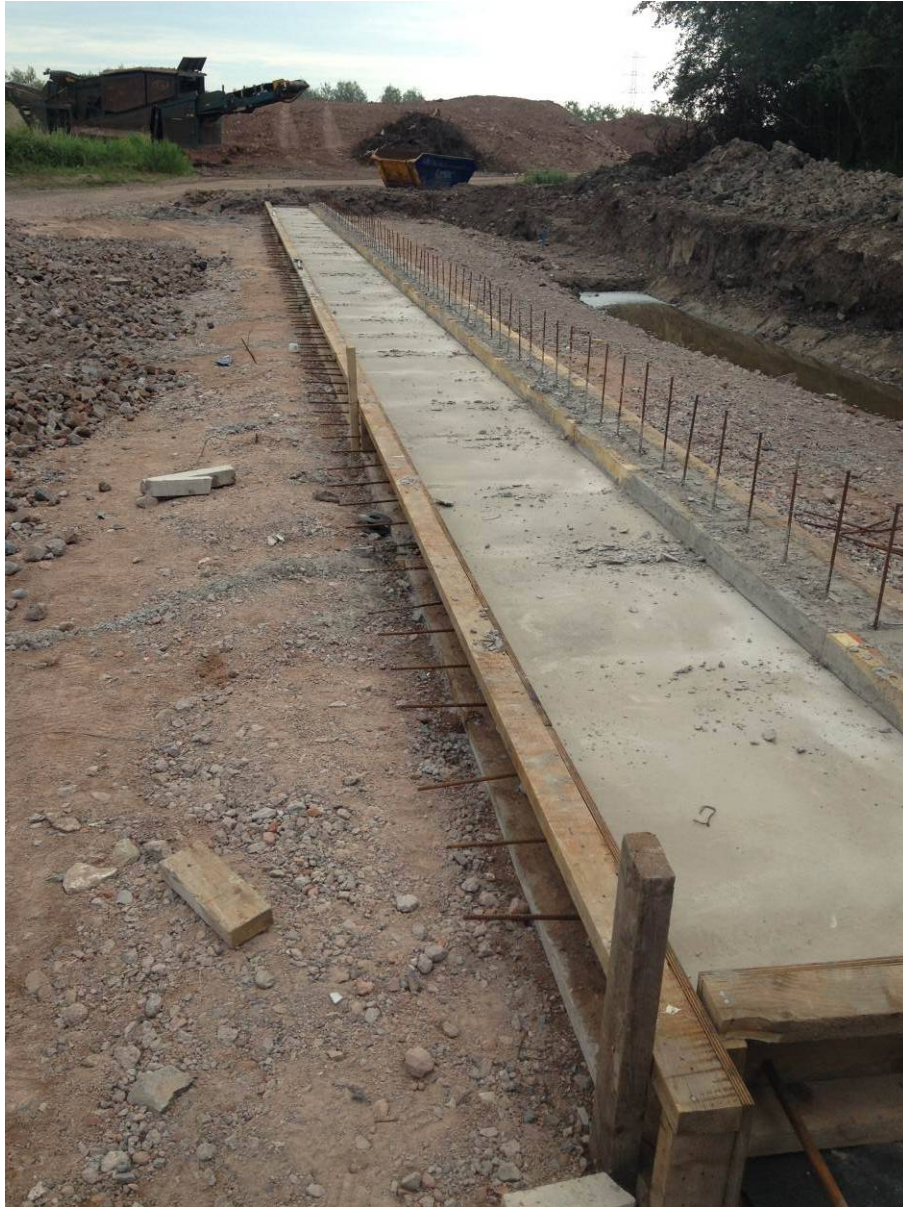
First section of concrete drainage channel
