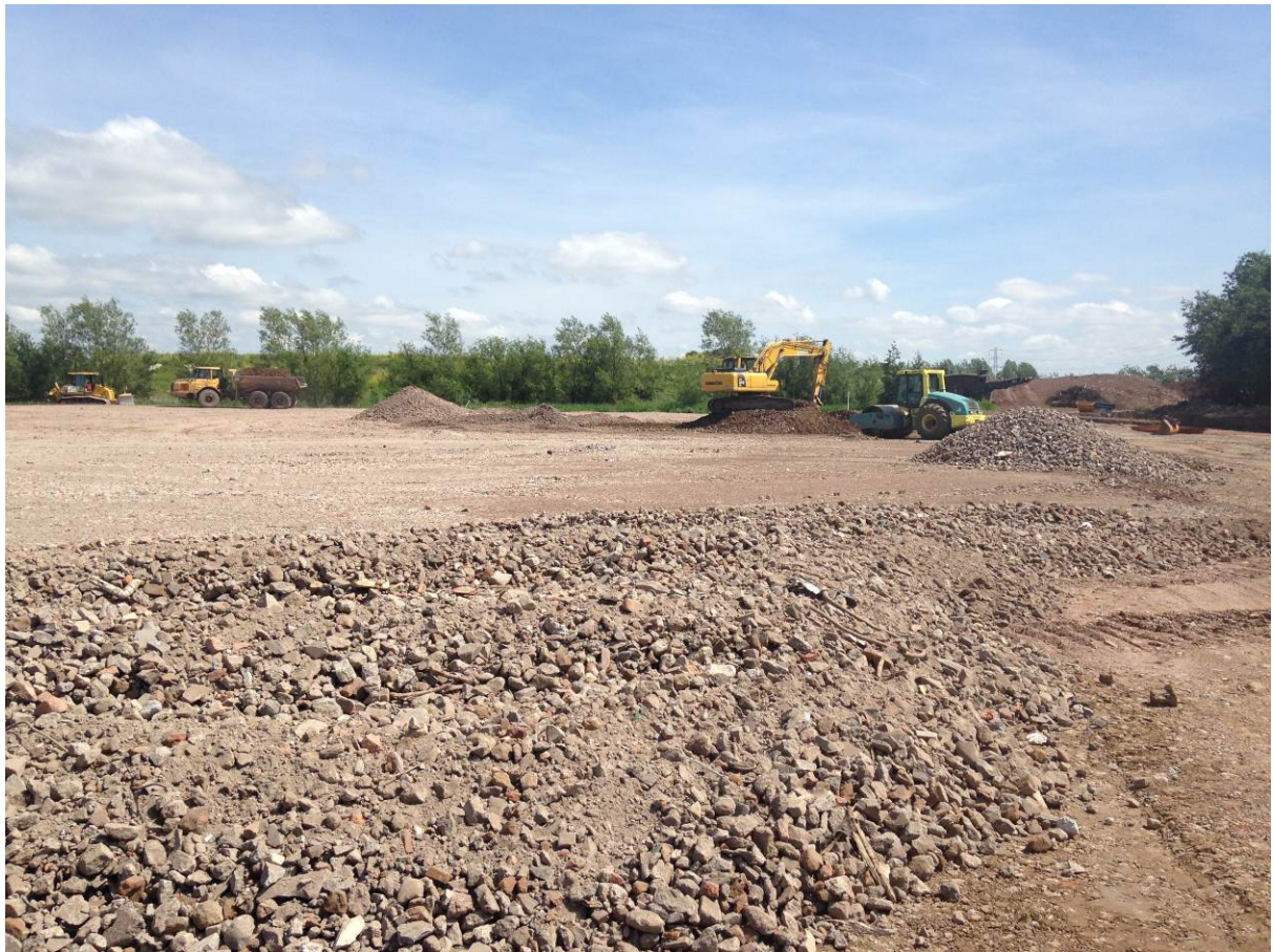
Edge of 300mm thick aggregate layer preparation
