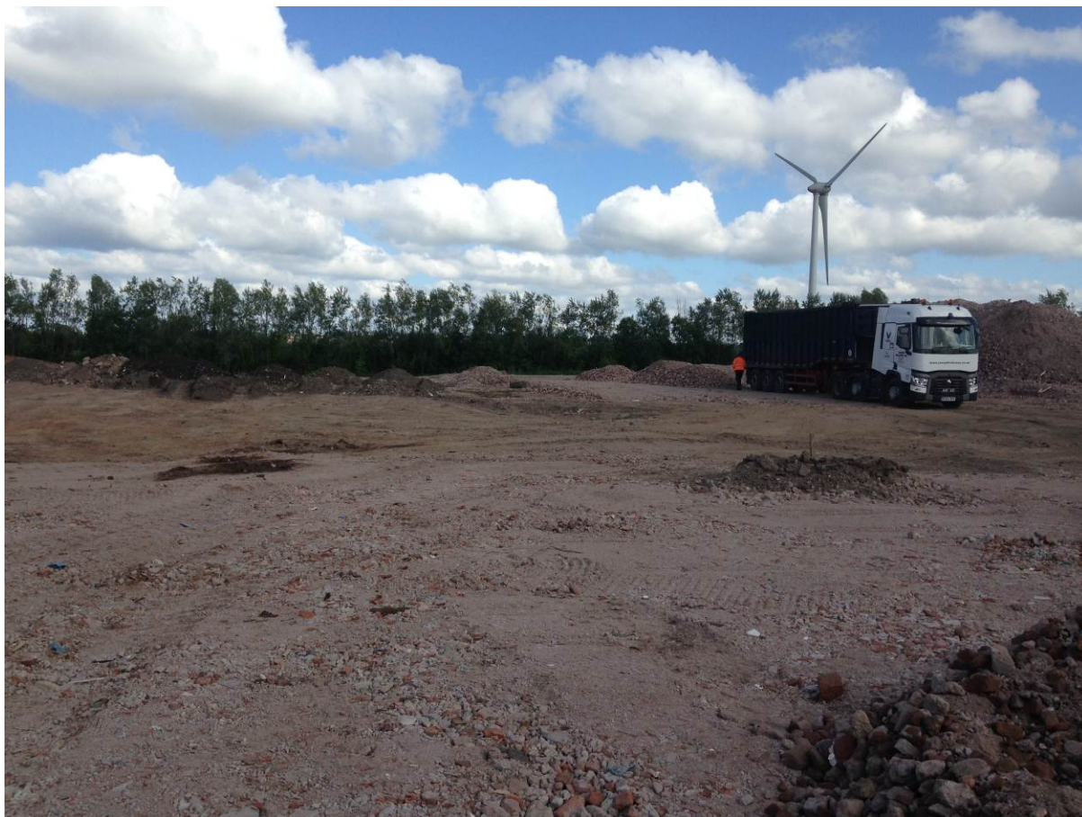
Delivery of aggregate to site
