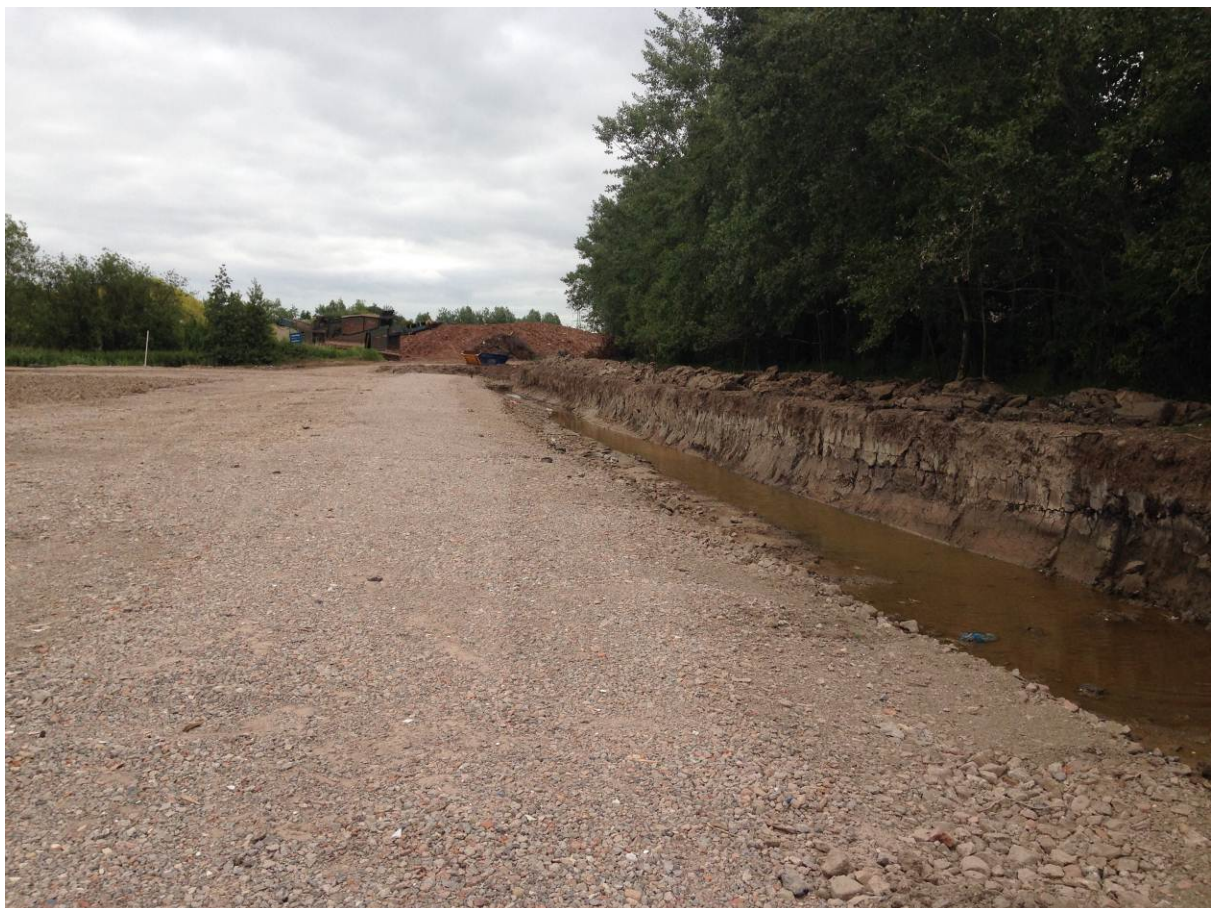
Southern edge of prepared area
