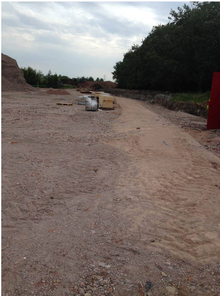
Dust layer prepared for Drainage Channel Construction
