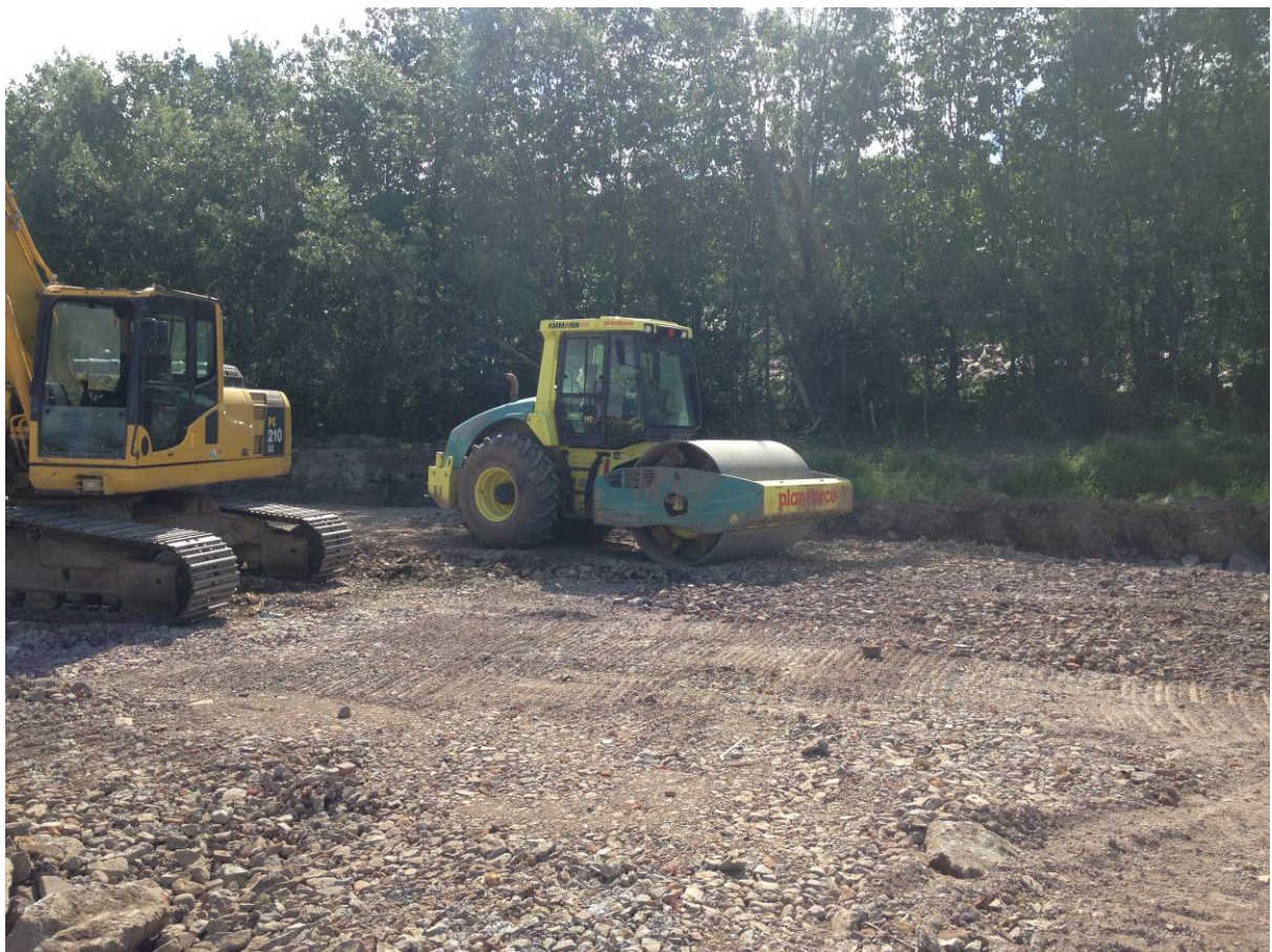
Final preparation of sub-grade for drainage channel
