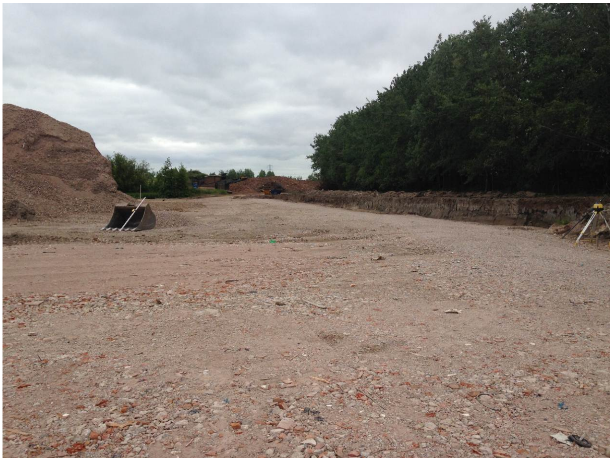
Aggregate stockpile and spinning laser setup
