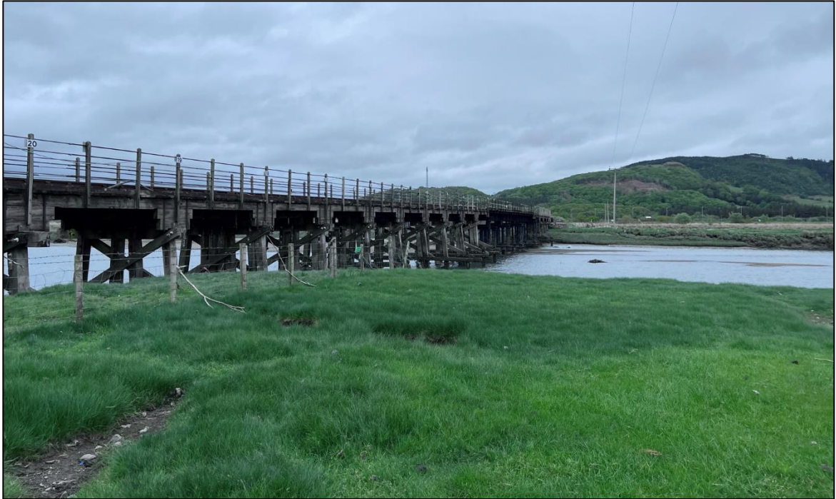
Figure 1: Dovey Junction Viaduct No.1 (From western shore).
