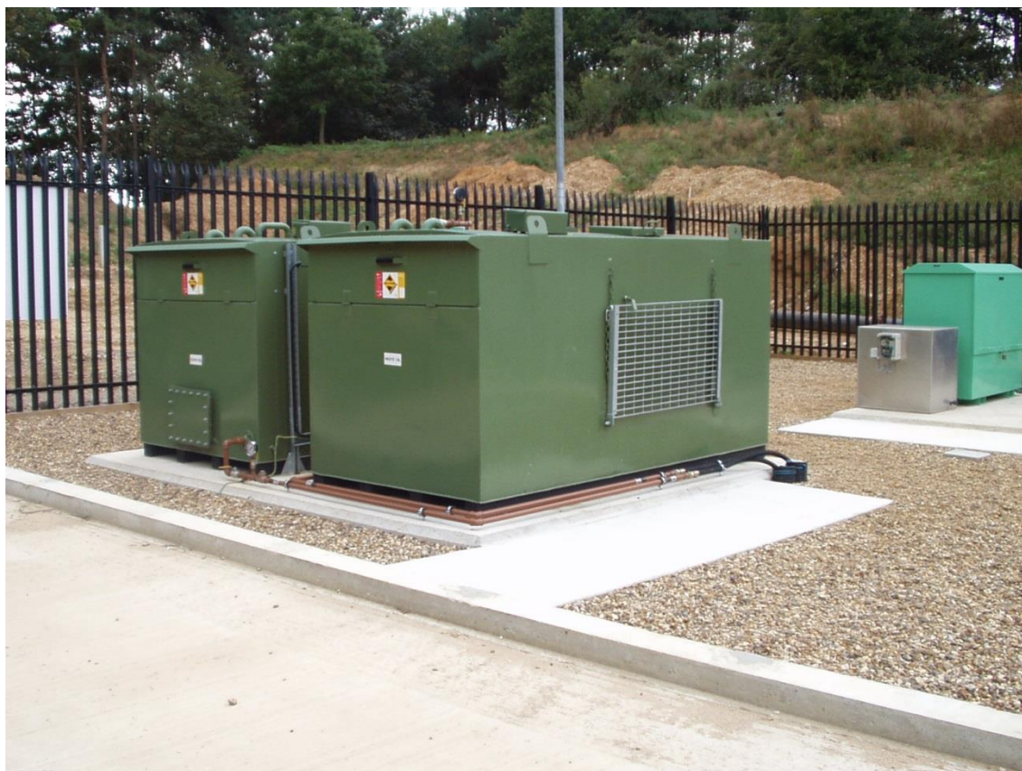
Figure 4.5 Typical bunded Oil Storage Tanks
