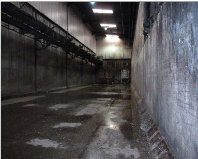
The photograph opposite was taken inside the RDF store. The store was empty following the change in status of the waste to energy plant. Water was evident on the floor of the store due to high humidity in the building.
