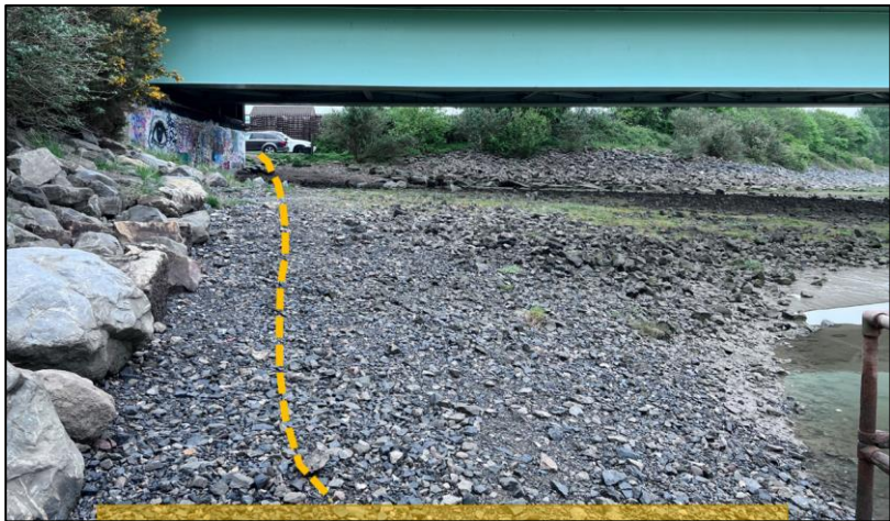
Figure 4: Access route to structure from laydown area.
