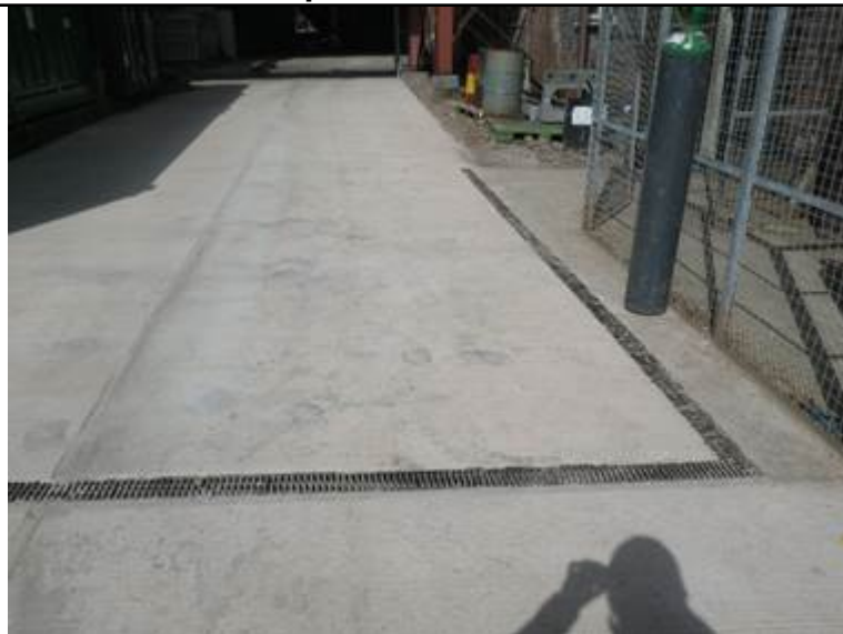
Photo 10: New impermeable surface
