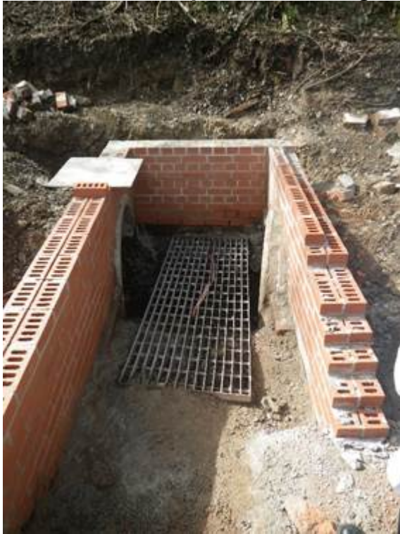
Photo 11: S30 in process of being re-built
