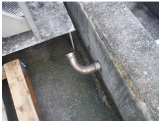
Photo 5 – redundant piping penetrating the bund
