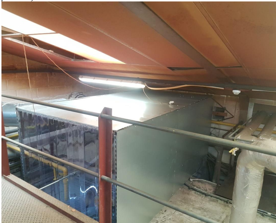
Fig 10 –New enclosure above kiln and extractor fans. (Red staining visible on roof due to previous emissions from kiln.)
