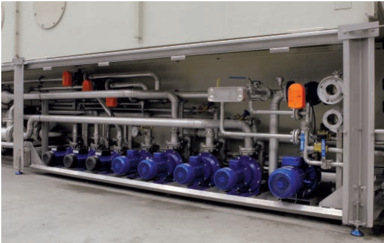
The skid-mounted utilities provide easy access and maintenance.
