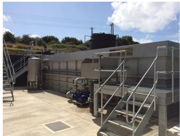
The DAF clarifier would be provided with a cover of 2.0 mm sheet stainless steel. It would be provided with inspection hatches and connections to direct vent gasses to an odour control filter.
