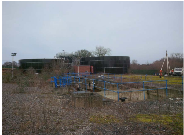
Plate 8. Effluent Treatment Plant – tanks and filter beds
