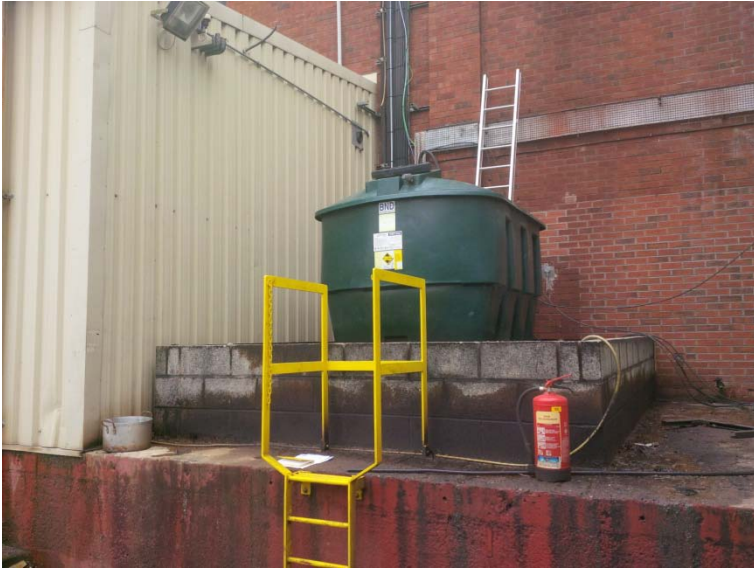
Plate 5. Fuel tank within concrete bund
