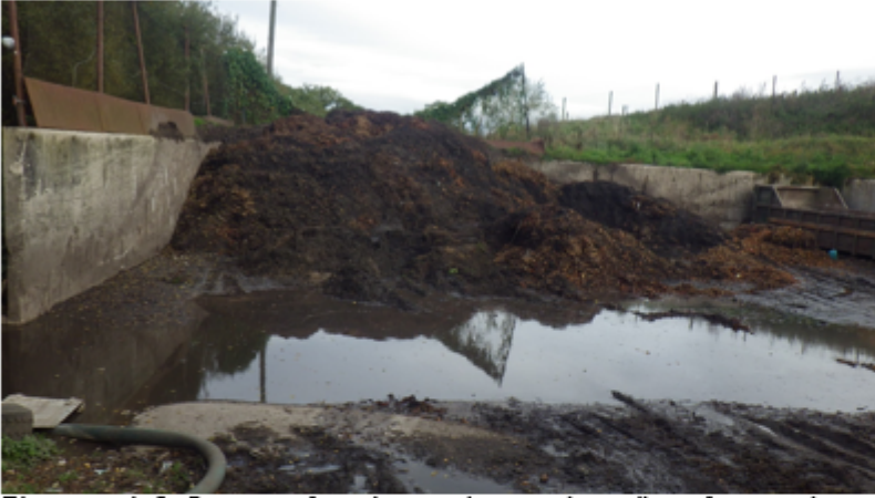
Photograph 3. Storage of road sweepings and ponding of contaminated water at the lower waste transfer pad.
