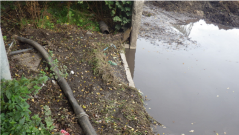
Photograph 4. Contaminated water from the lower transfer pad ponding and evidence of previous emission to ground
