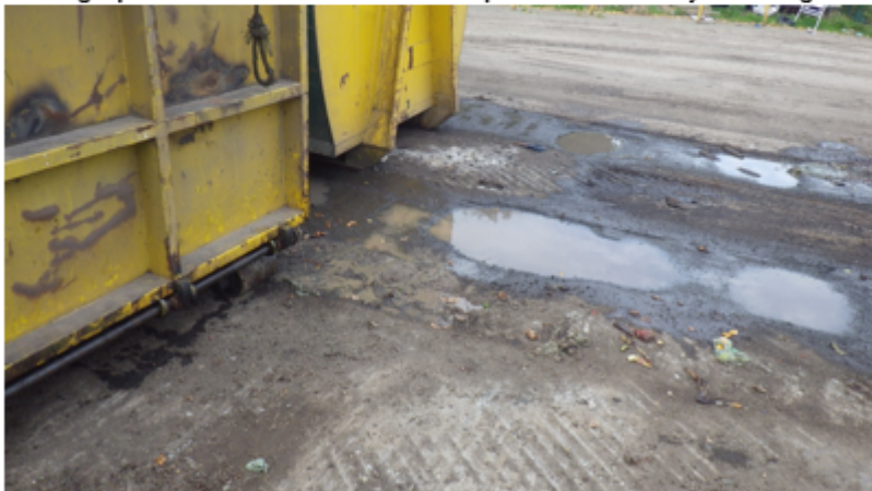
Photograph 8. Ponding of effluent from the food waste storage.
