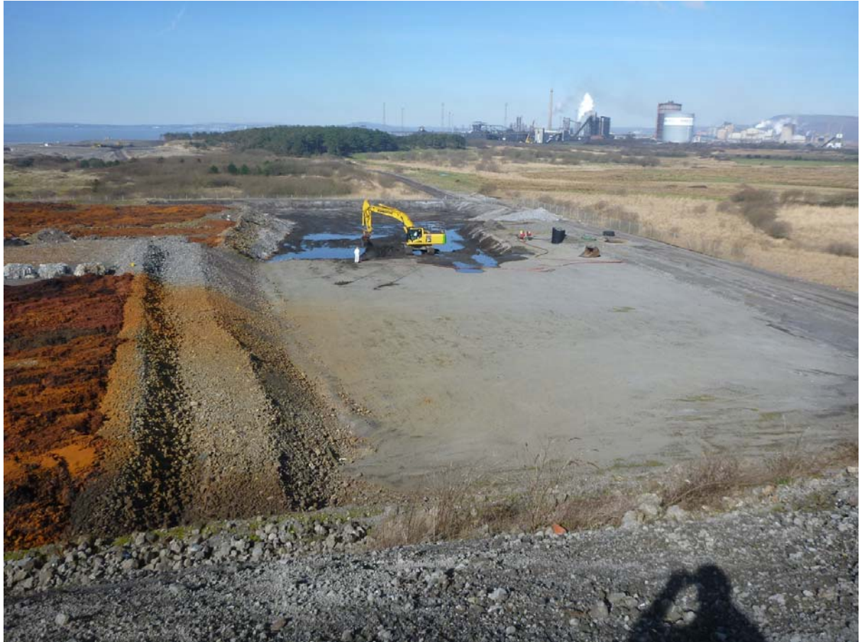
Fire wastes being carefully removed from the Non Hazardous cell for transfer top the Hazardous landfill
