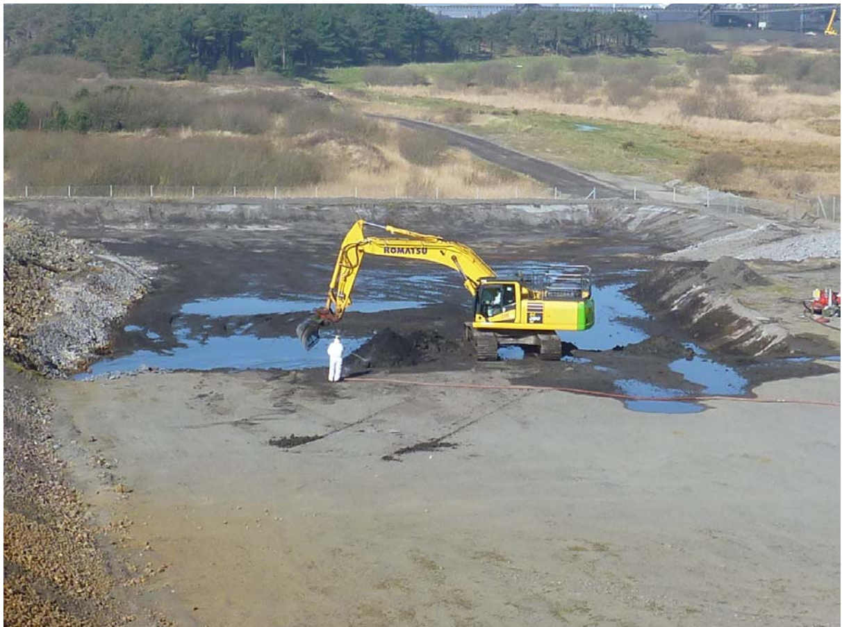
Fire wastes being carefully removed from the Non Hazardous cell for transfer top the Hazardous landfill
