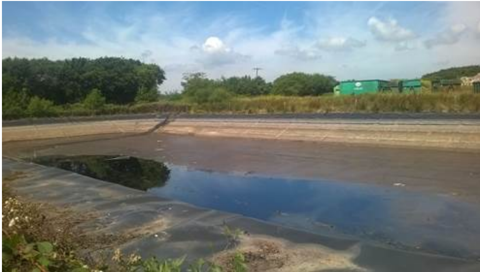
Pic 2. Site main leachate holding lagoon. At the time of the inspection the temperature was hot. No rain had occurred for several days resulting in the lagoon being nearly empty.
