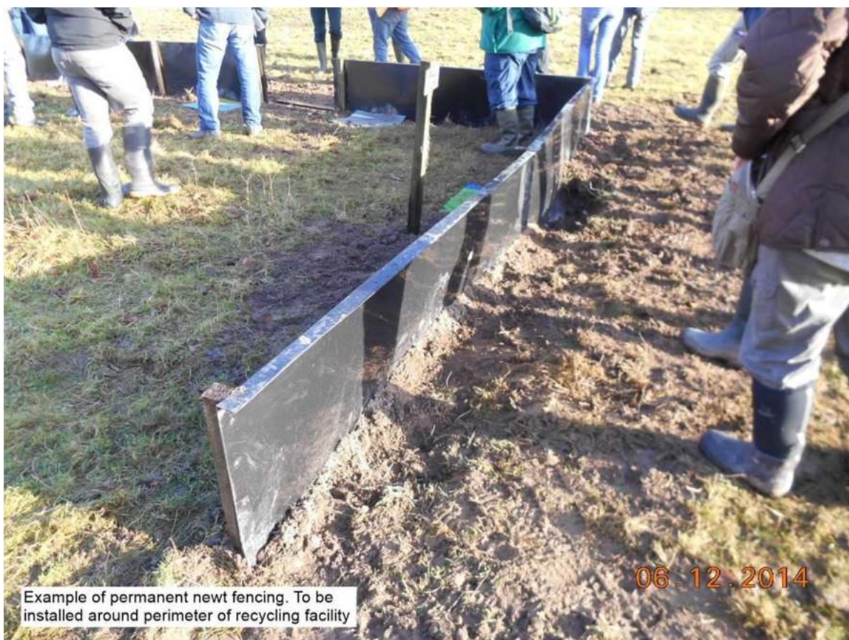
Permanent 3-4mm newt fence panel showing underground section and underlap.
