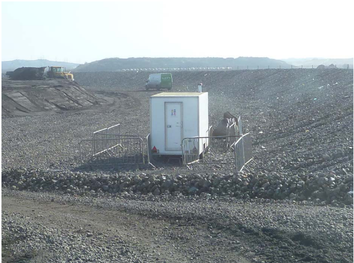
Asbestos decontamination unit.
