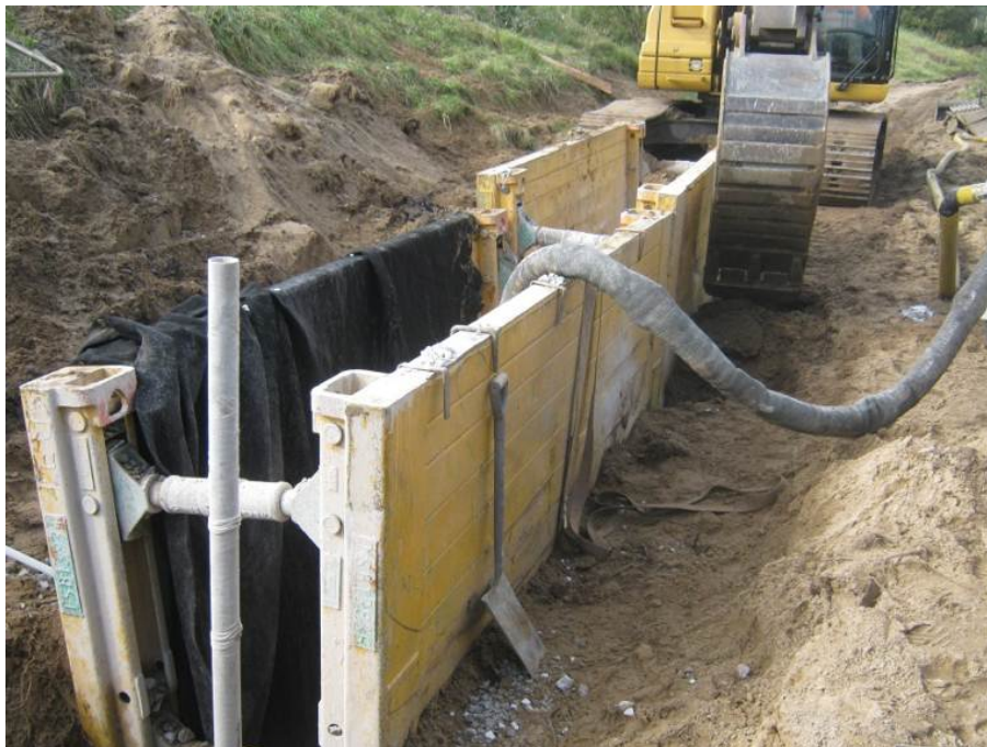
Construction of Recharge Trench
