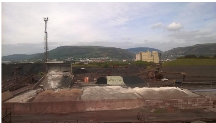
Sinter fines bed being started by the machine at centre-right
