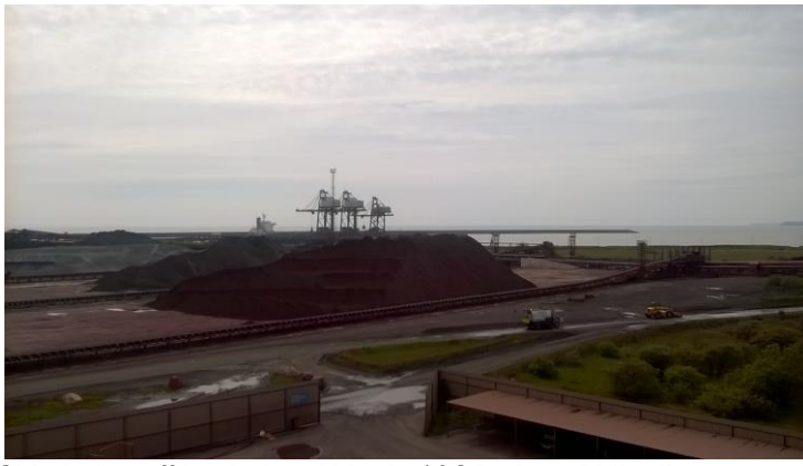
Ship being off loaded and Yards 1&2 in the middle distance. The road is being swept by the white vehicle.
