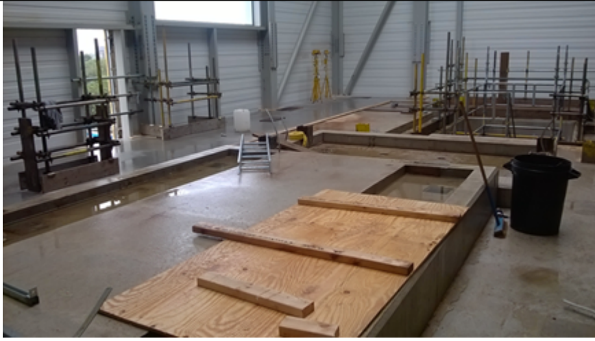
Photo 4 – Turbine plinth within turbine hall
