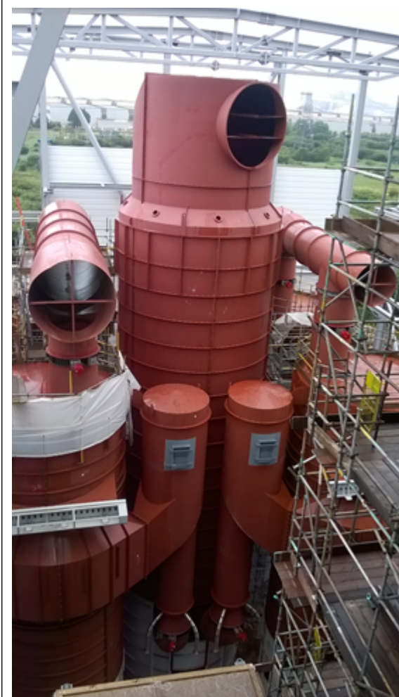
Photo 3 – Section of flue gas treatment system (65m stack)
