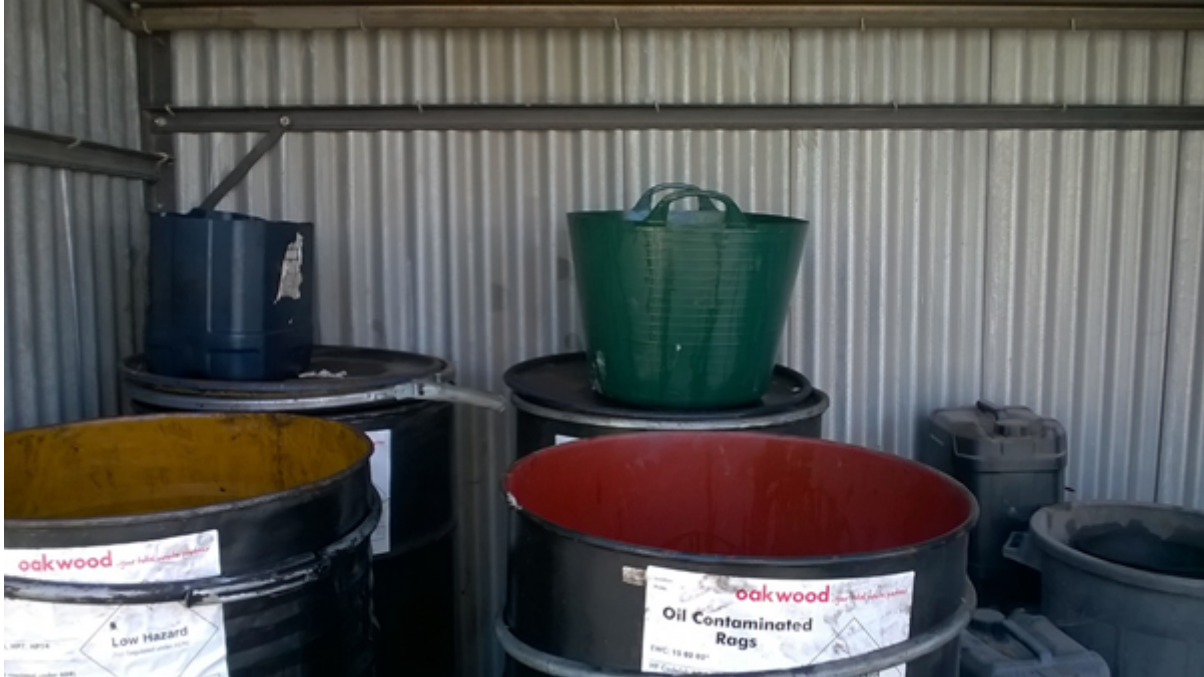
Pic 2. Chemicals/Oil store. Open vessels seen containing waste materials need to have lids attached when not in use to reduce the risk of pollution and fire.
