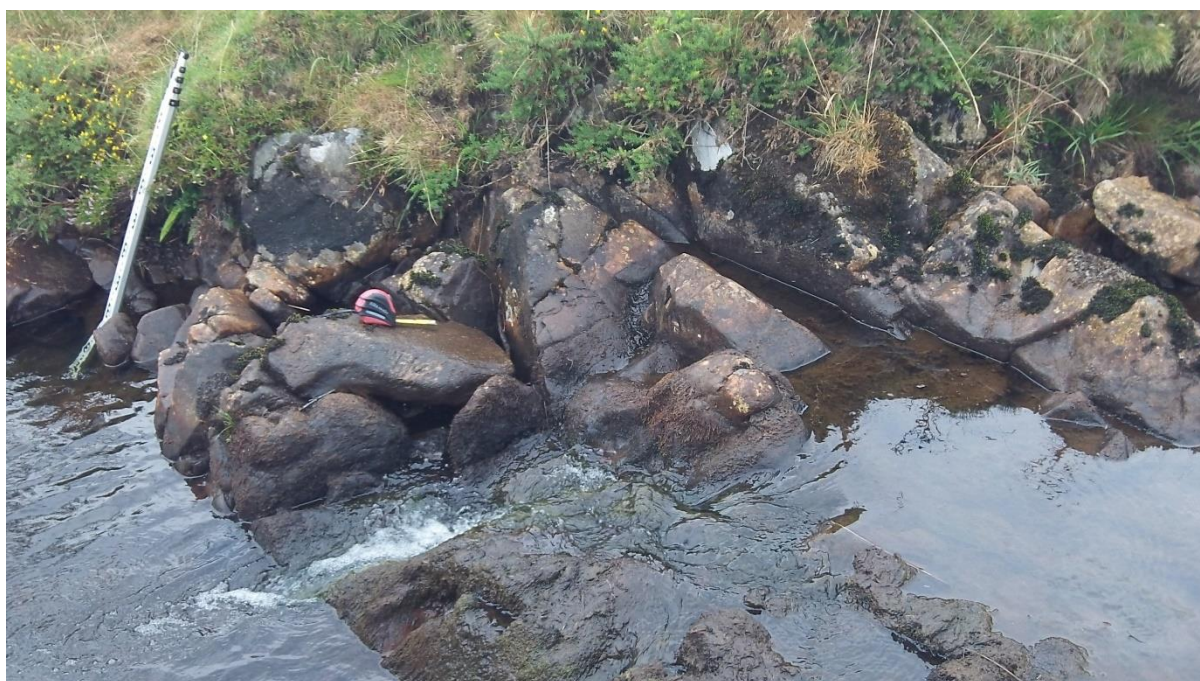
Intake A - Right Bank
