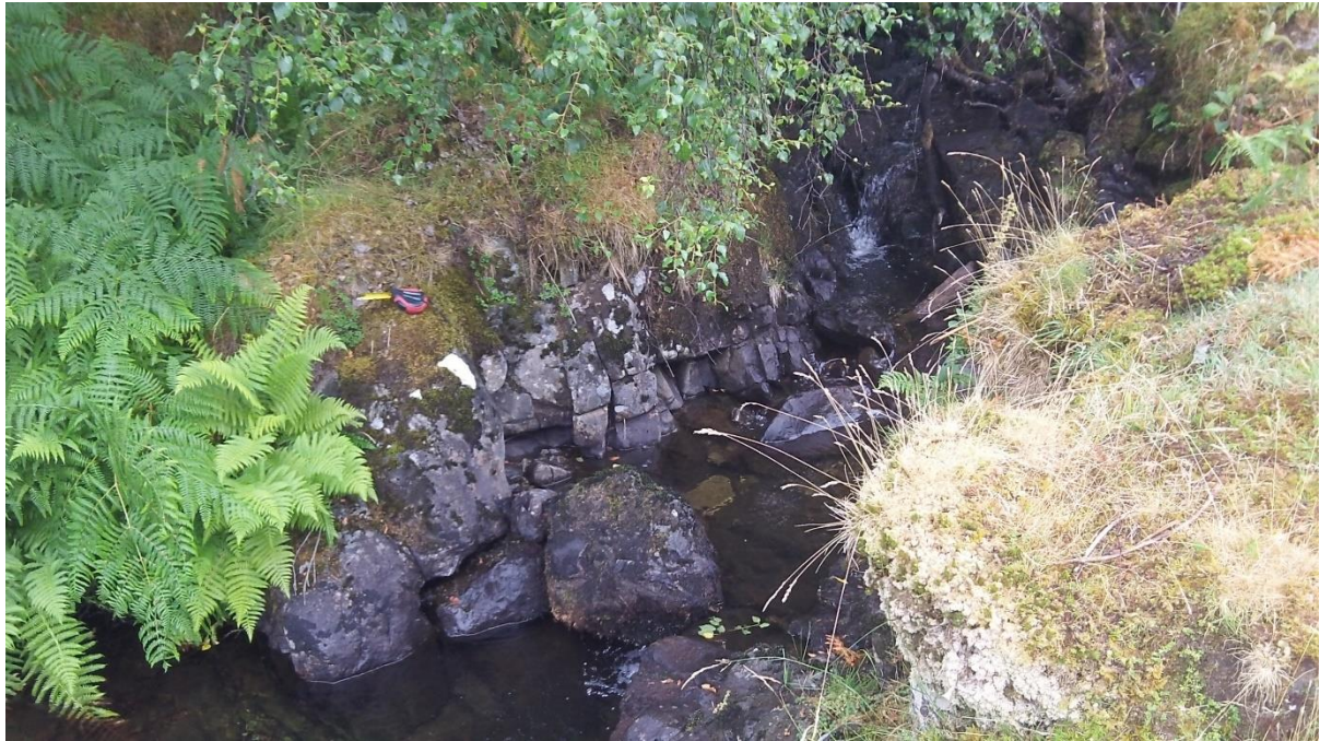
Intake B - Right Bank
