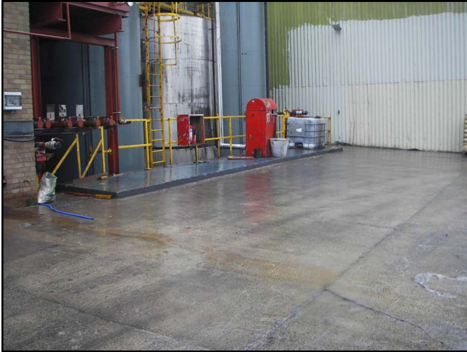
Picture 9 – Installation of Containment Bund required to ensure the capture of potential spills.
