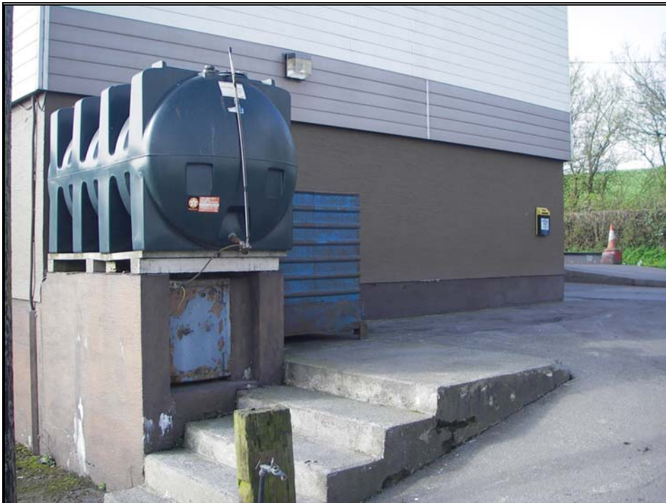
Picture 10 – Installation of Fuel Tank Bund with 110% Capacity to ensure the capture of potential spills.
