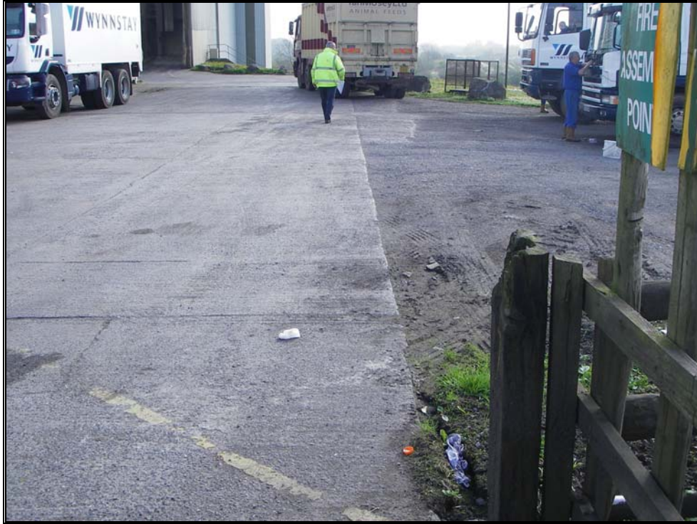
Picture 11 – Installation of ACO surface water drainage required to ensure the on-site capture and treatment of surface waters.
