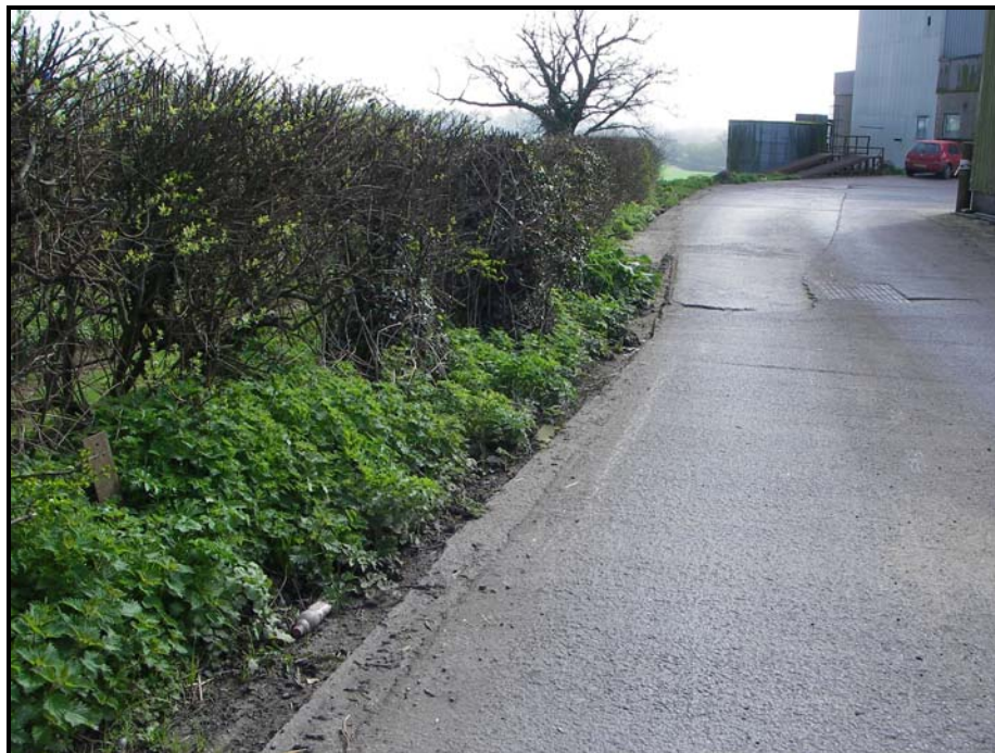
Picture 2 – Installation of Surface Kerb required to ensure the on-site containment and treatment of surface waters.
