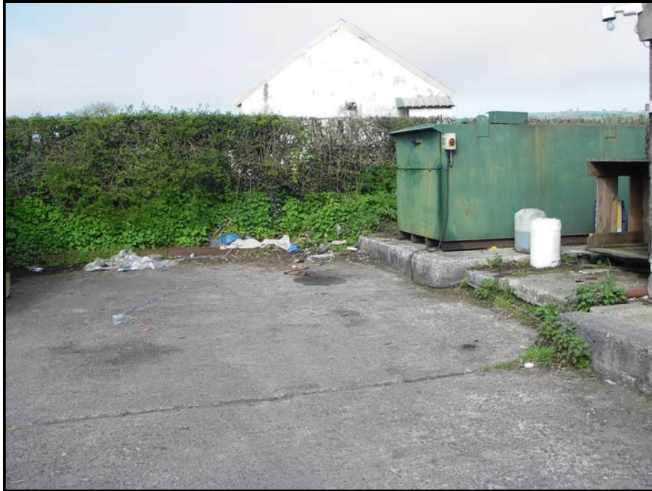
Picture 1 – Installation of ACO Drainage required to ensure capture and treatment of possible fuel spills.
