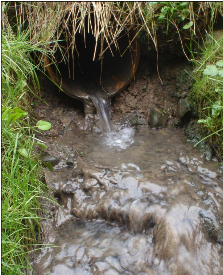
Photo 1: Sewage fungus discharging from main office septic tank overflow outfall.
