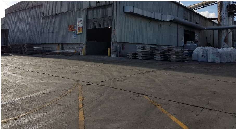
Figures 5: Sealed Infrastructure
