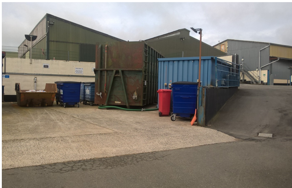
Photo 1 - Portable tank (green Gileskip portable liquid storage tank) located within waste storage area
