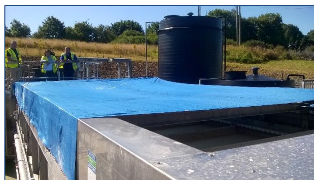
Photographs showing the DAF unit which has now been fitted with a tarpaulin cover to minimise odour
