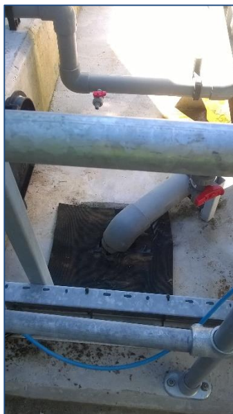
Portable drain covers in use around the sludge tanks and sludge thickening unit
