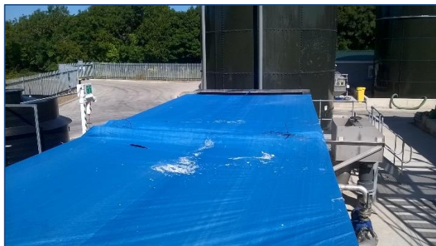
Photographs showing the DAF unit which has now been fitted with a tarpaulin cover to minimise odour
