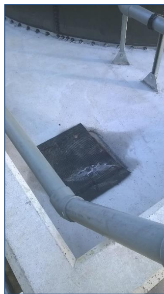
Portable drain covers in use around the sludge tanks and sludge thickening unit
