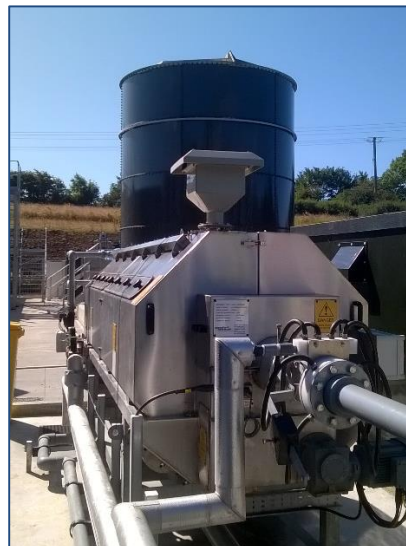
Examples of carbon filters fitted to the sludge tanks and sludge thickening unit
