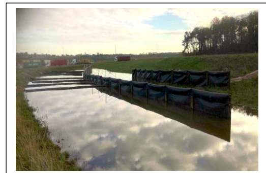
Images of static impermeable silt curtains to manage flow pathways and floating treatment curtains
