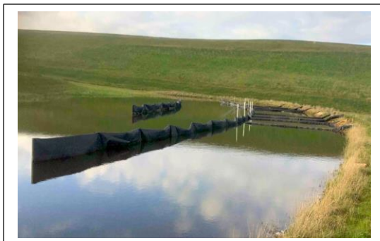
Images of static impermeable silt curtains to manage flow pathways and floating treatment curtains
