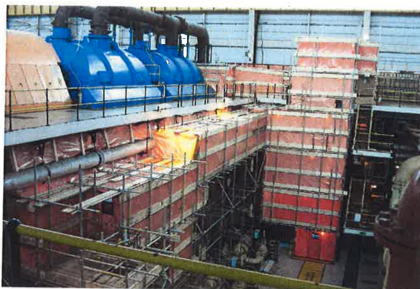
Photograph 3 Turbine Hall Asbestos Removal at Hinkley Point A Power Station
