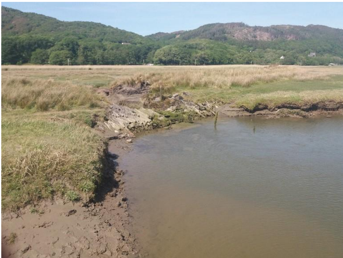
Looking north - extent of saltmarsh adjacent to the breach
