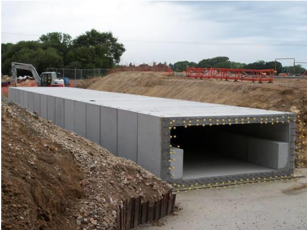
Fig. 5 Example of precast culvert under construction
