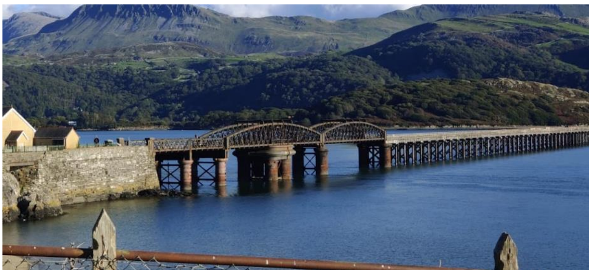
Fig. 2: Railway Bridge, looking East
