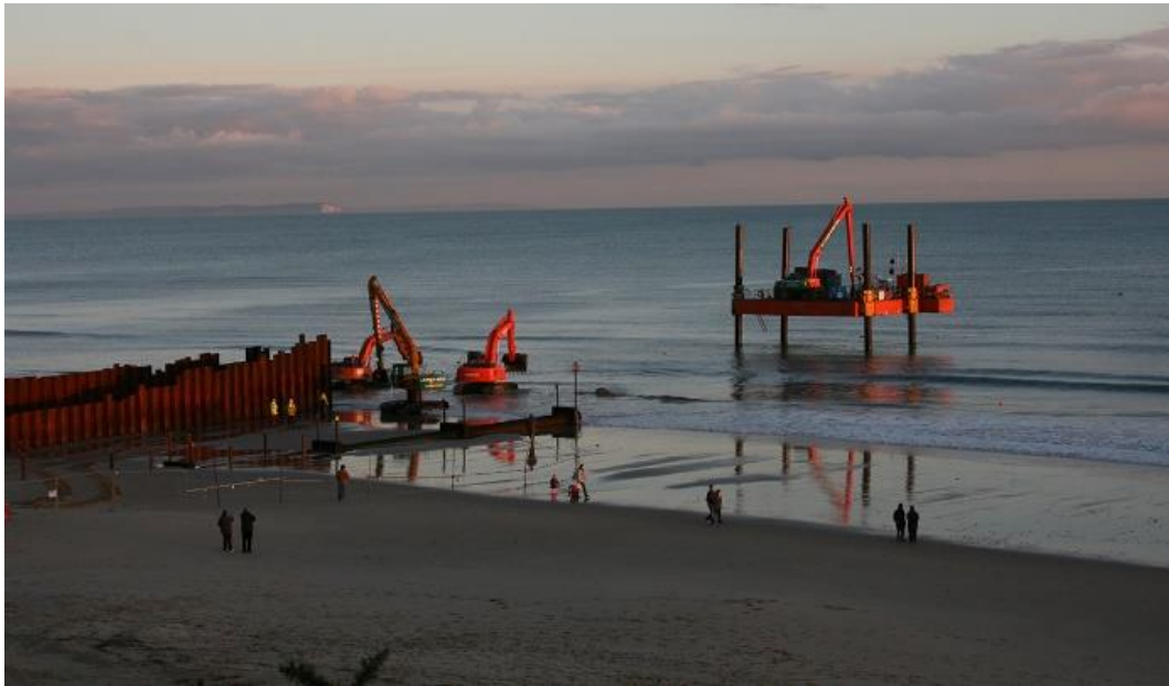
Fig. 4 Example of Jack-Up rig and Marine Sheet Piling
