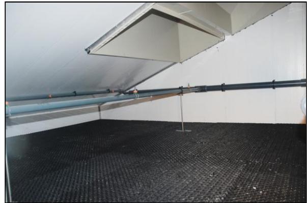
Figure 14: Filter pack with sprinkler pipes
