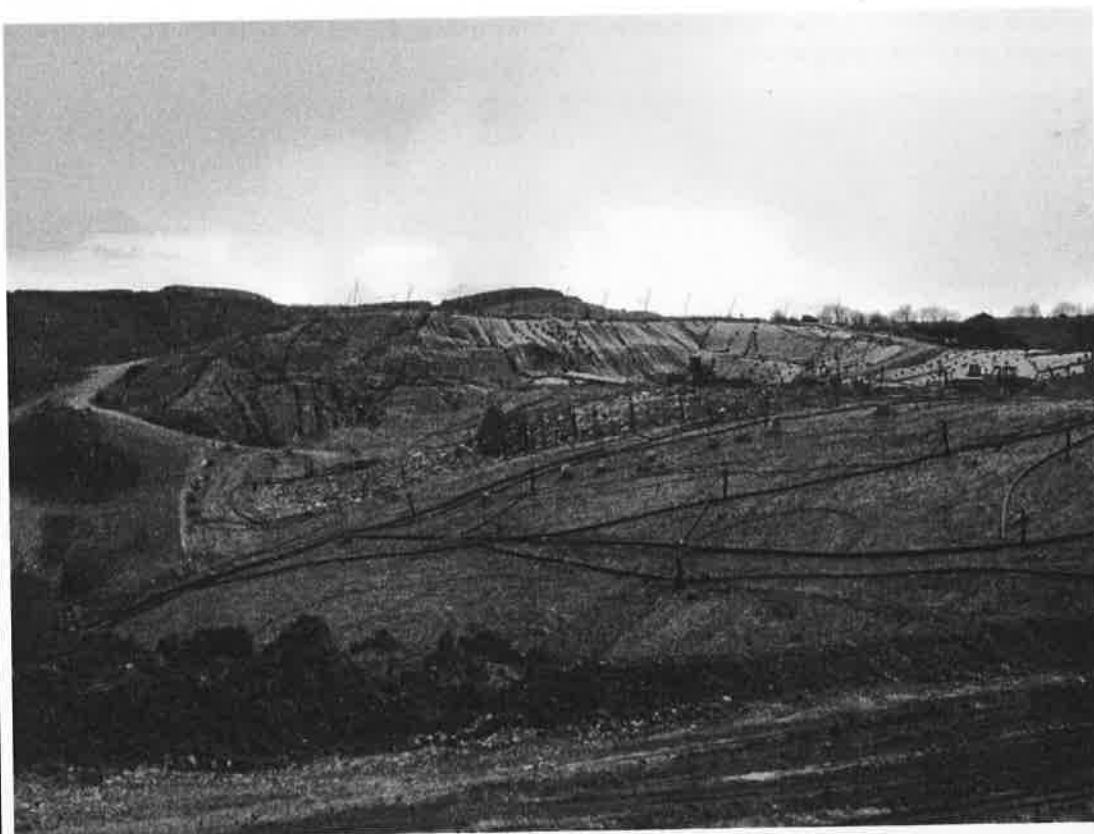
Capping and gas infrastructure on Northern flank of Phase 3A North:
