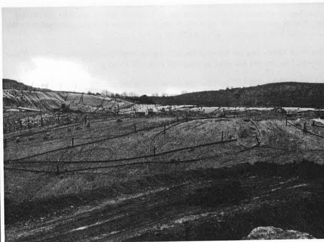
Capping and gas infrastructure on Northern flank of Phase 3A North:
