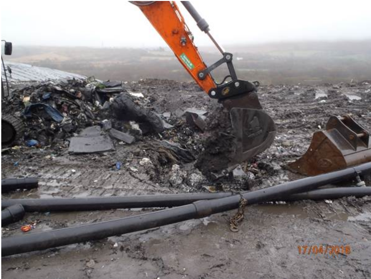
Photographs of gas infrastructure installation & tipping face:
