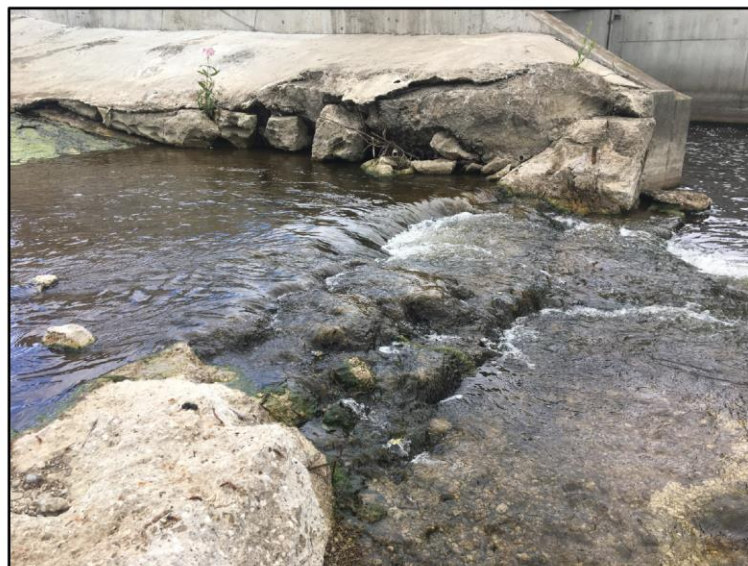
Photo showing Northern Pre-Barrage following removal of 4m section.
