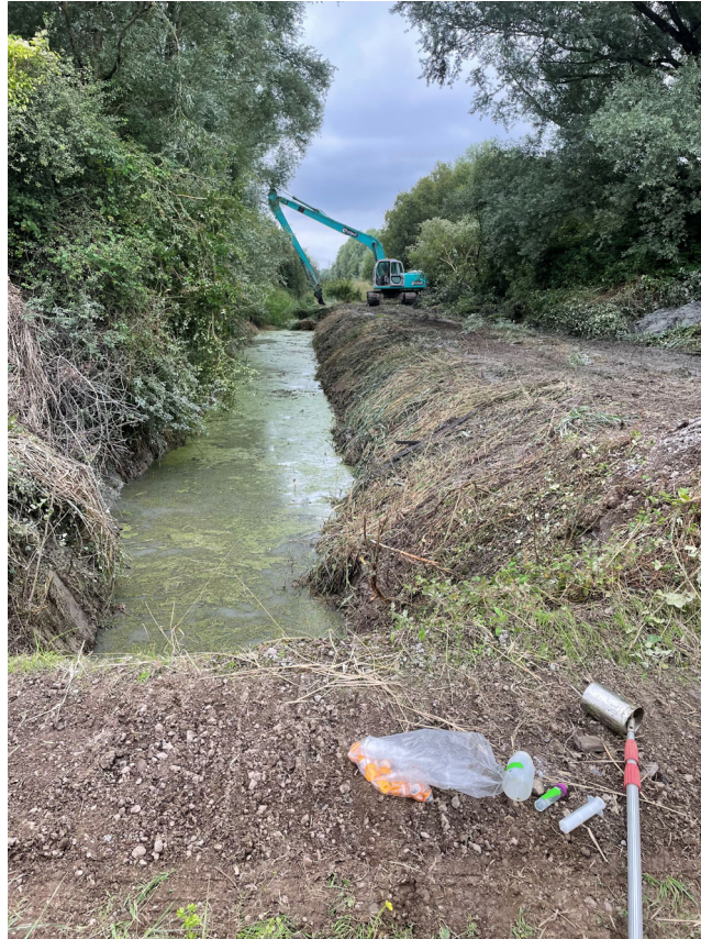
Plate 6-2 Ditch maintenance during August 2021 sampling
