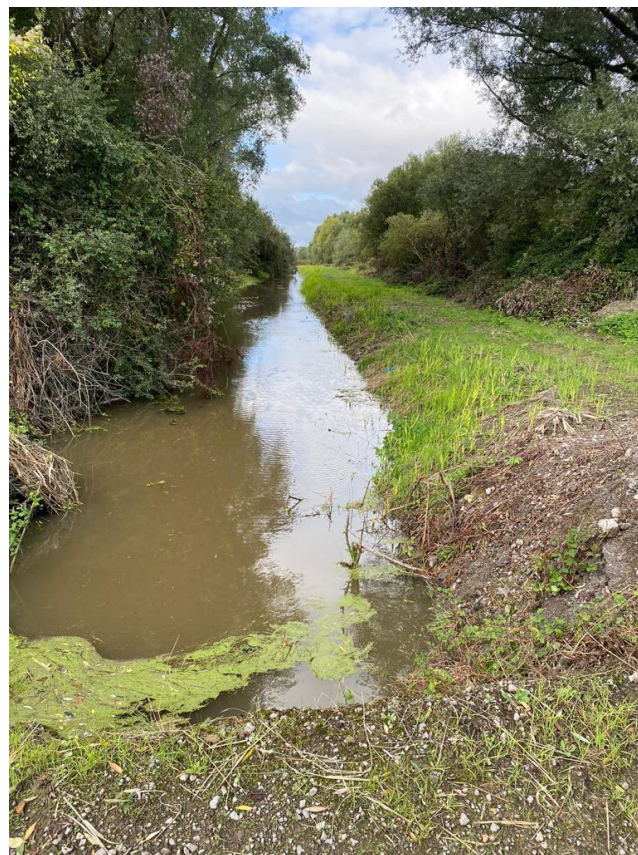
Plate 6-3 Raised surface water levels in October 2021
