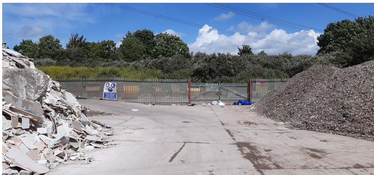
Photo 2 - Some windblown debris located at GD Environmental
