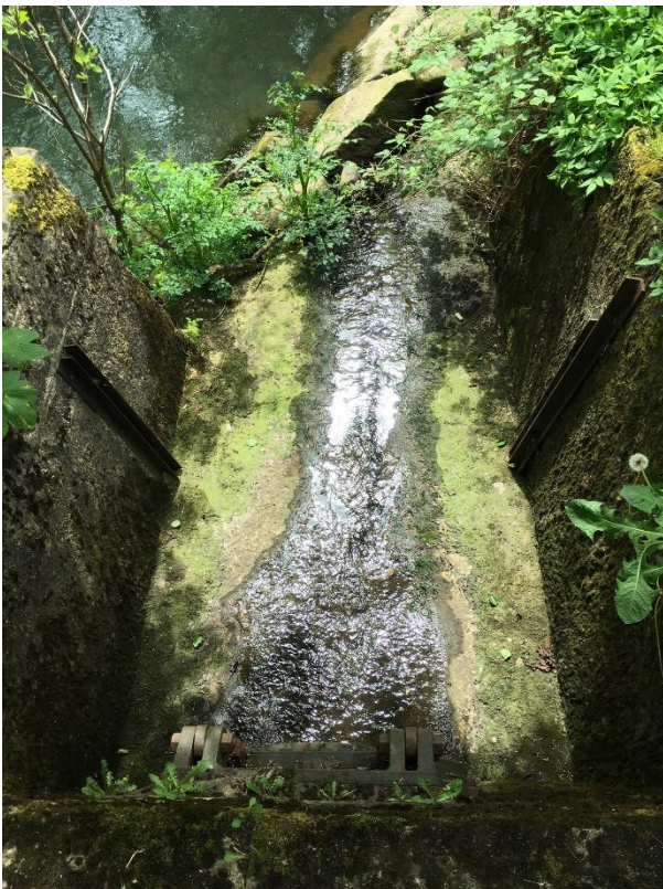
Discharge point flap and plinth
