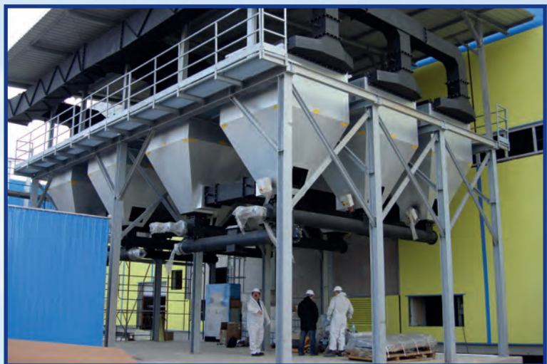
HTMC12(400) under construction.
