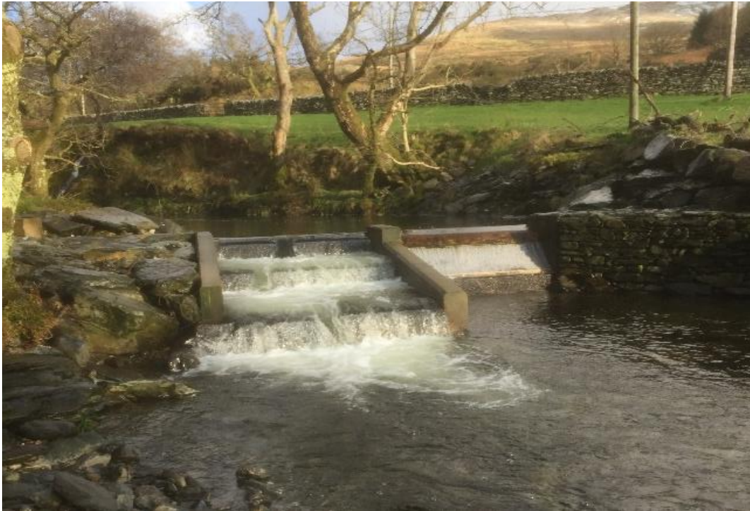
Figure 1-3. The Coanda intake structure and fish pass for the existing HEP scheme on the Afon Colwyn.
