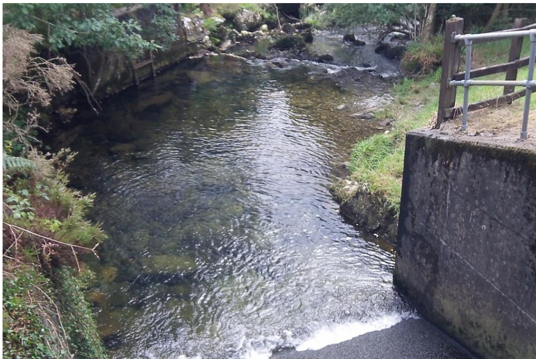
Figure 2-2. The base of the gauging weir looking towards the rock cascade, showing the presence of a deeper resting pool towards the left bank.
