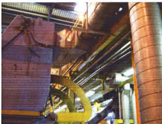
Rear of shredder unit, showing exhaust ventilation ducting
