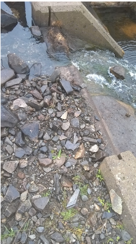
Photo 2: Gravel build up on the compensation flow section possibly minimising the flow
