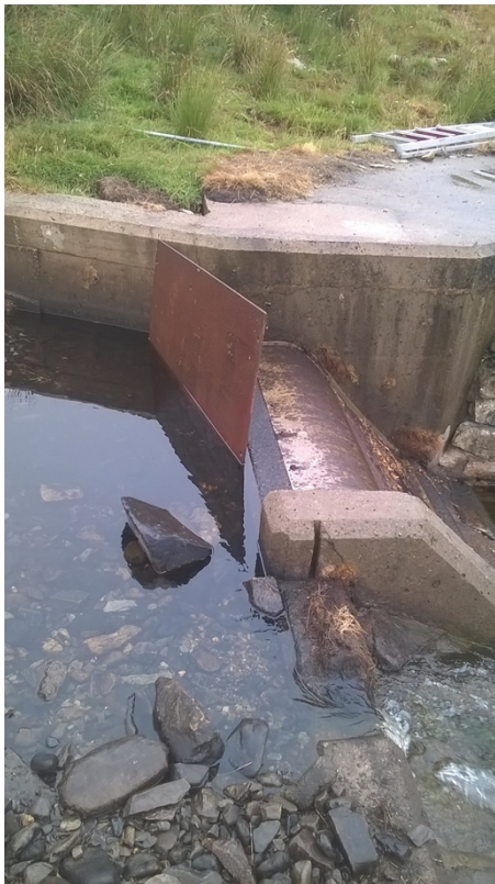
Picture 4: Showing the blocking of the abstraction notch to ensure a 50/50 split flow.
