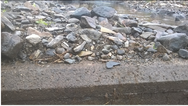
Picture 3: Gravel and stone build artificially raising the level of the compensation flow which will reduce the compensation flow proportionally to the abstraction notch flow.
