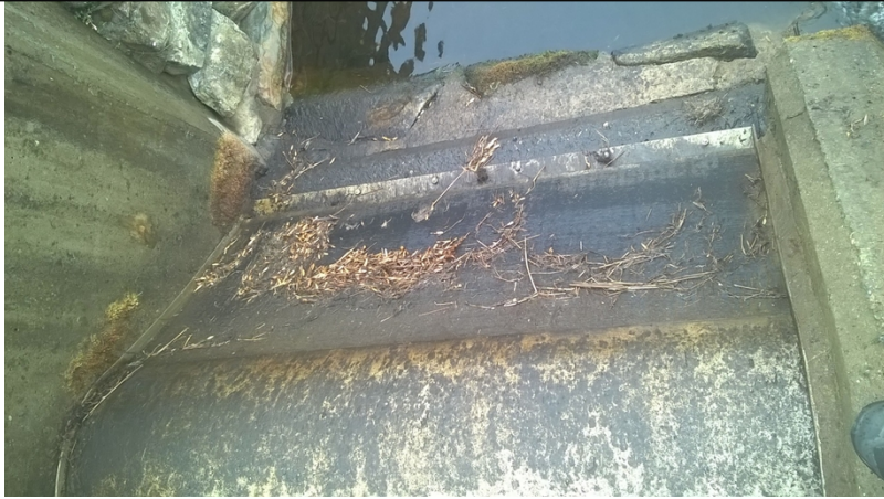
Picture 5: Appropriate sized screen and screen spacing.
